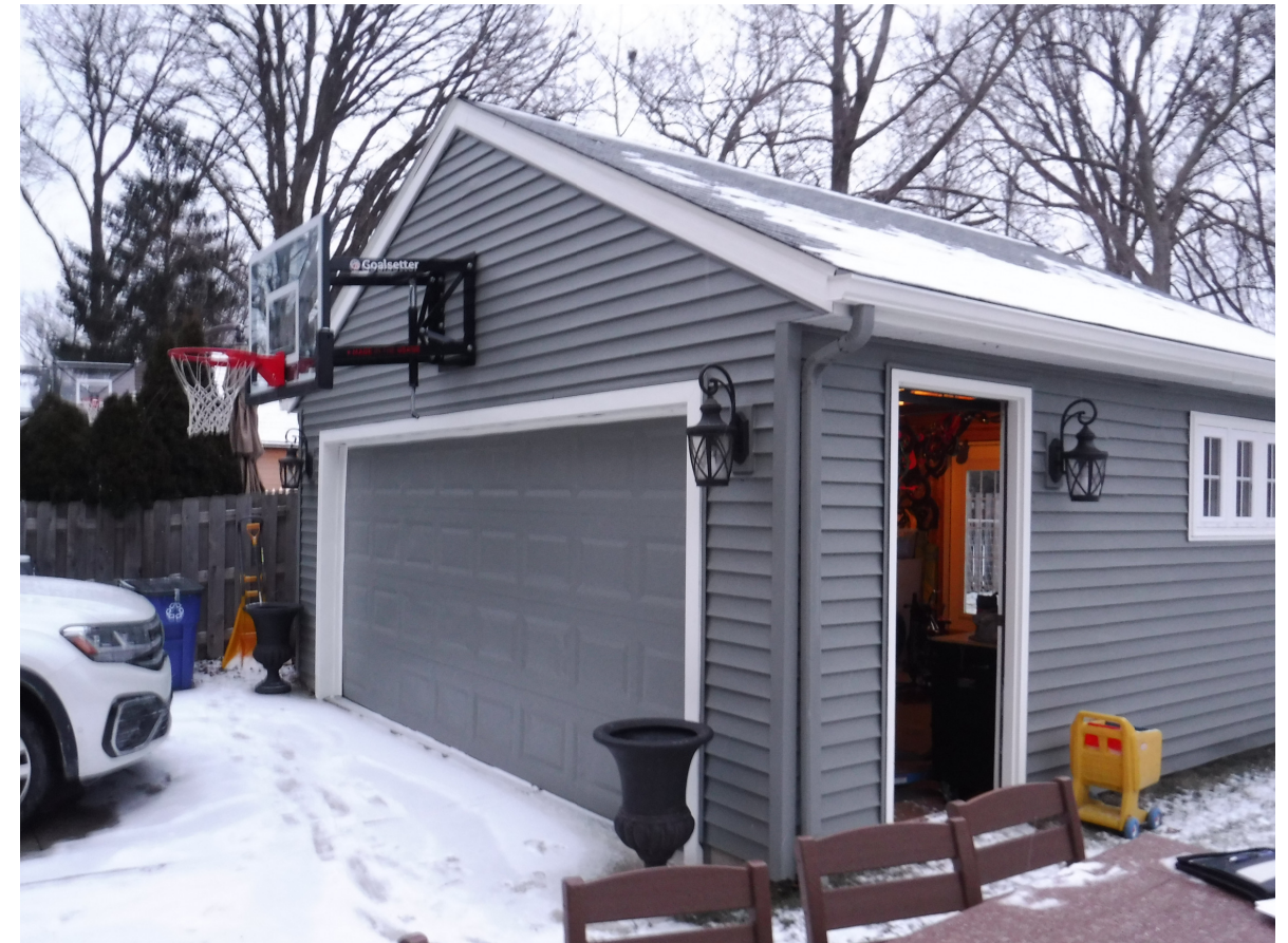
EXISTING CONDITIONS PHOTO VIEWING SOUTHEAST N.T.S.
