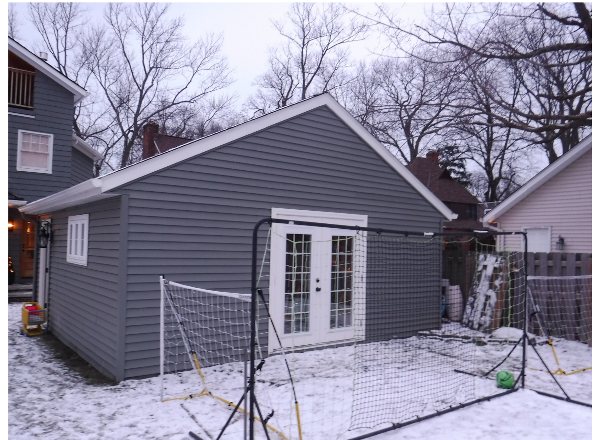
EXISTING CONDITIONS PHOTO VIEWING NORTHEAST N.T.S.
