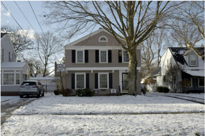
EAST/FRONT VIEW - PROJECT PROPERTY 2858 GASSER BOULEVARD
