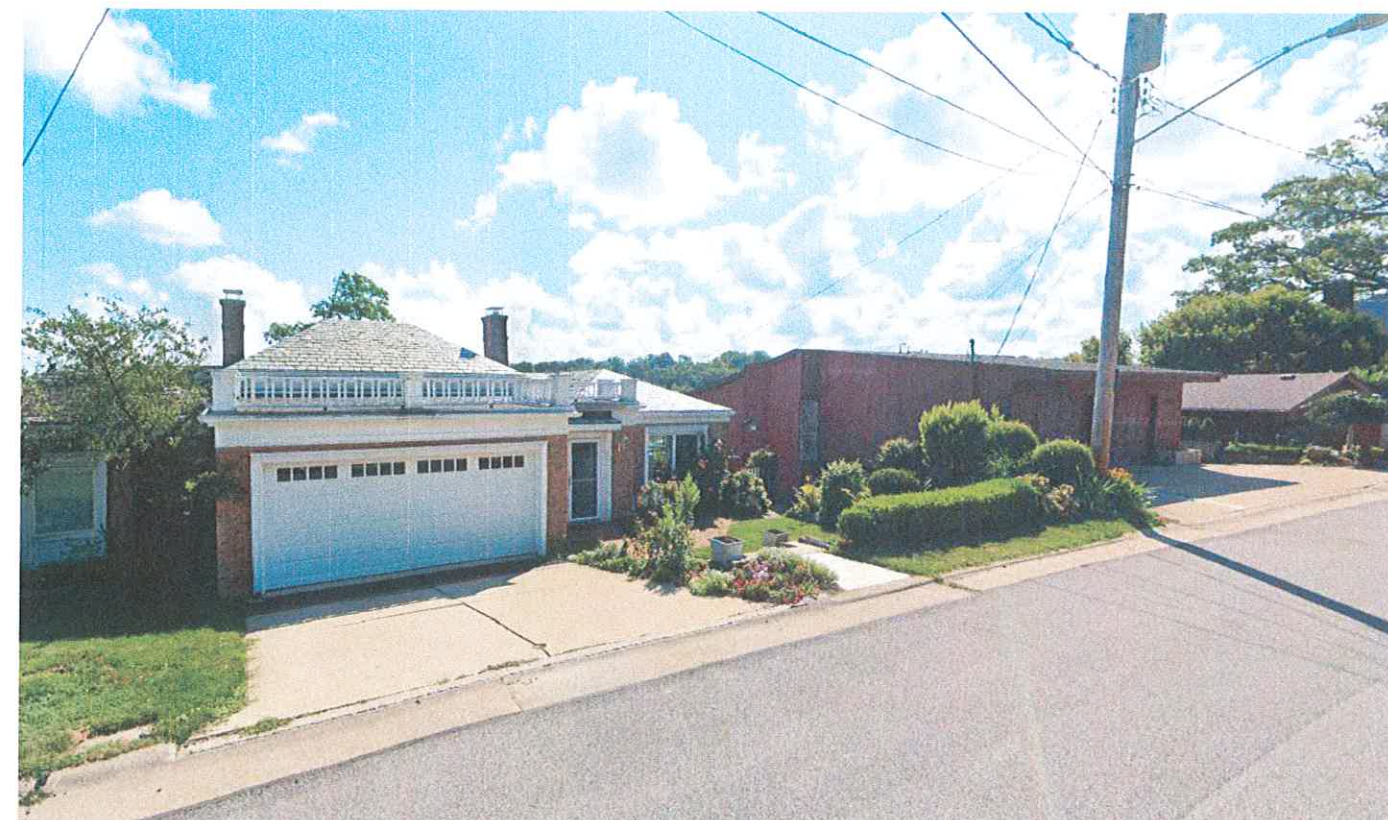
Neighboring Residences (Frazier Drive)
