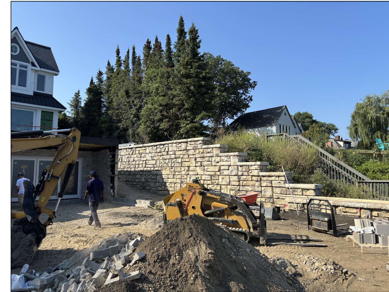
EXISTING VIEW OF RETAINING WALL
