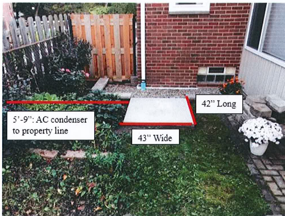
Figure 5 (Variance 1): Measurements for the proposed location of the AC condenser. Northwest corner of the rear-yard.
