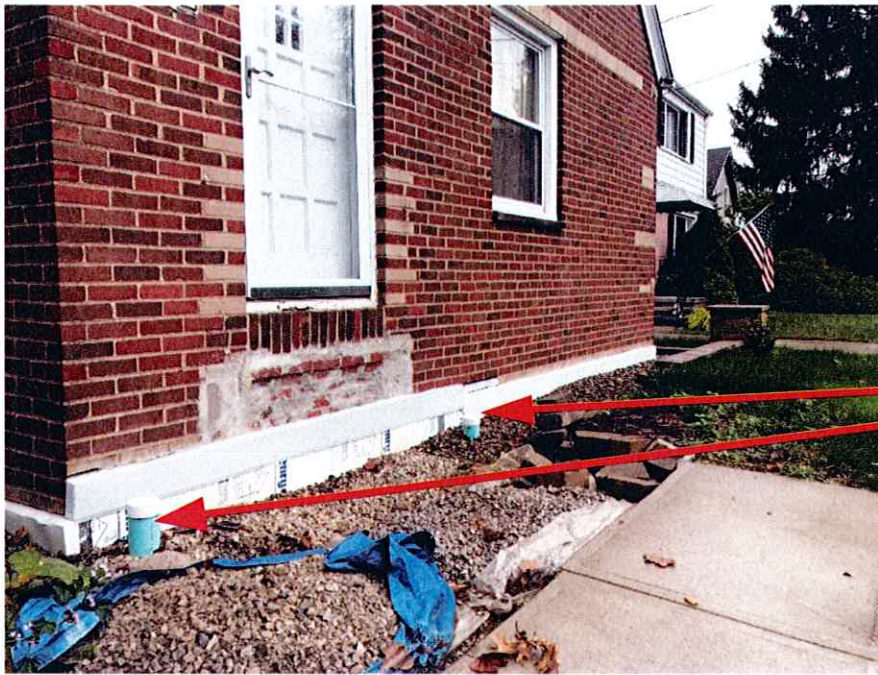
Figure 12 (Variance 2): Location of the downspout drain pipes for the front stoop gable roof.
