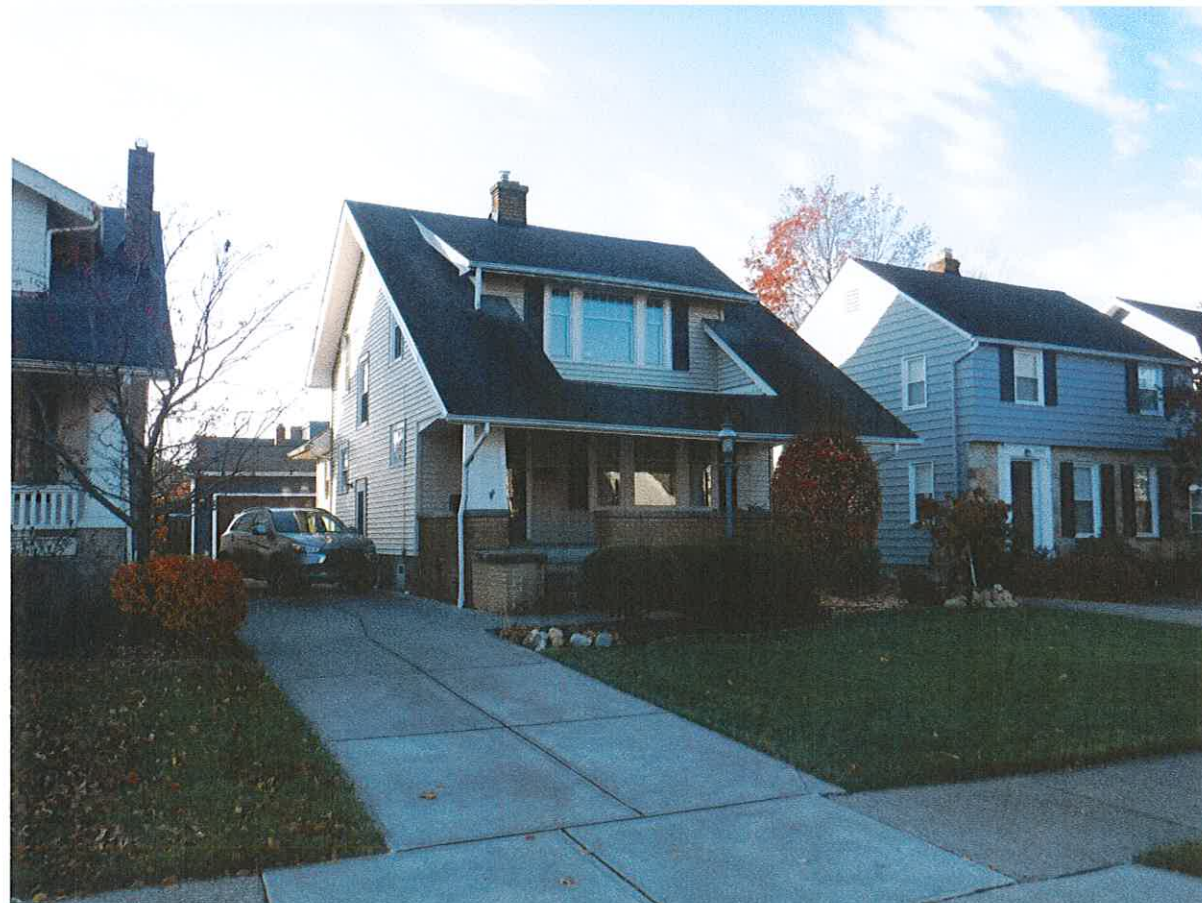
FRONT OF EXISTING HOME VIEWING SOUTHWEST
