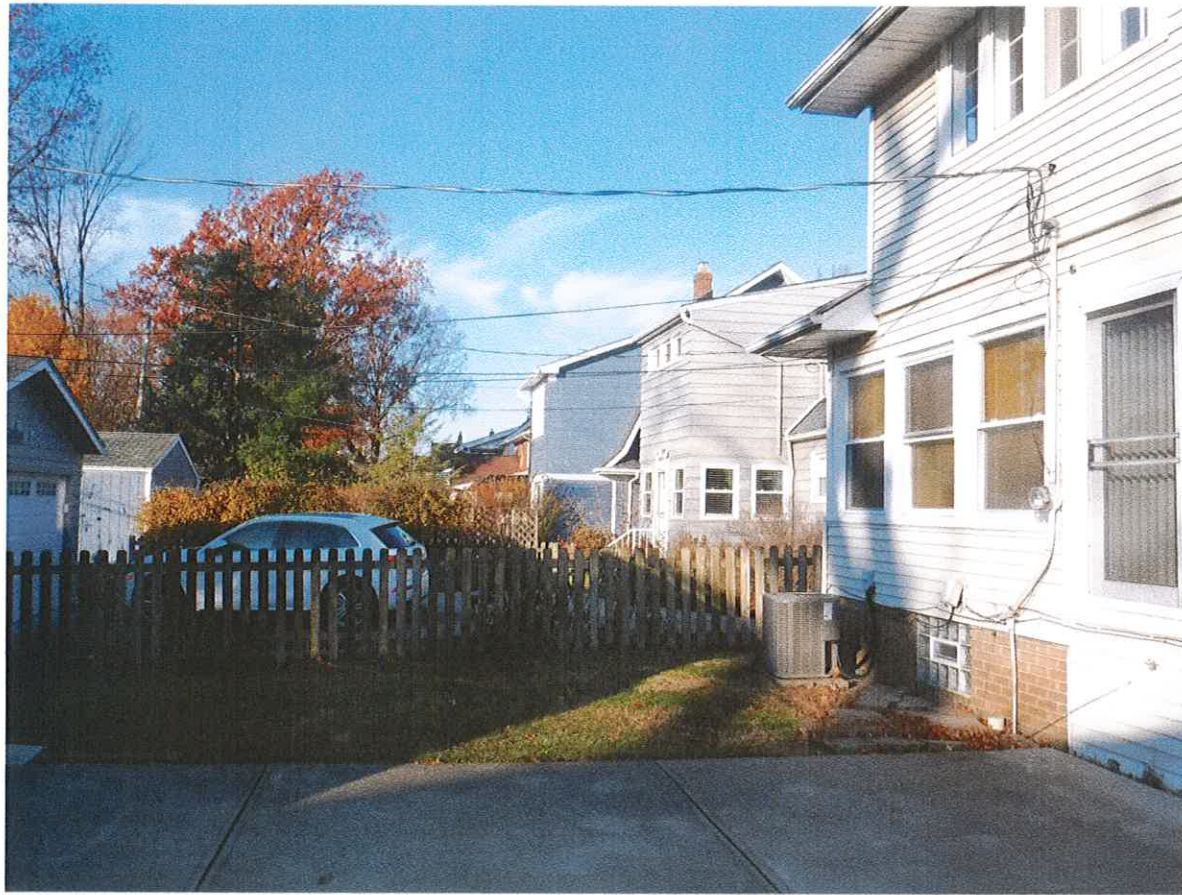
REAR OF EXISTING HOME VIEWING WEST
