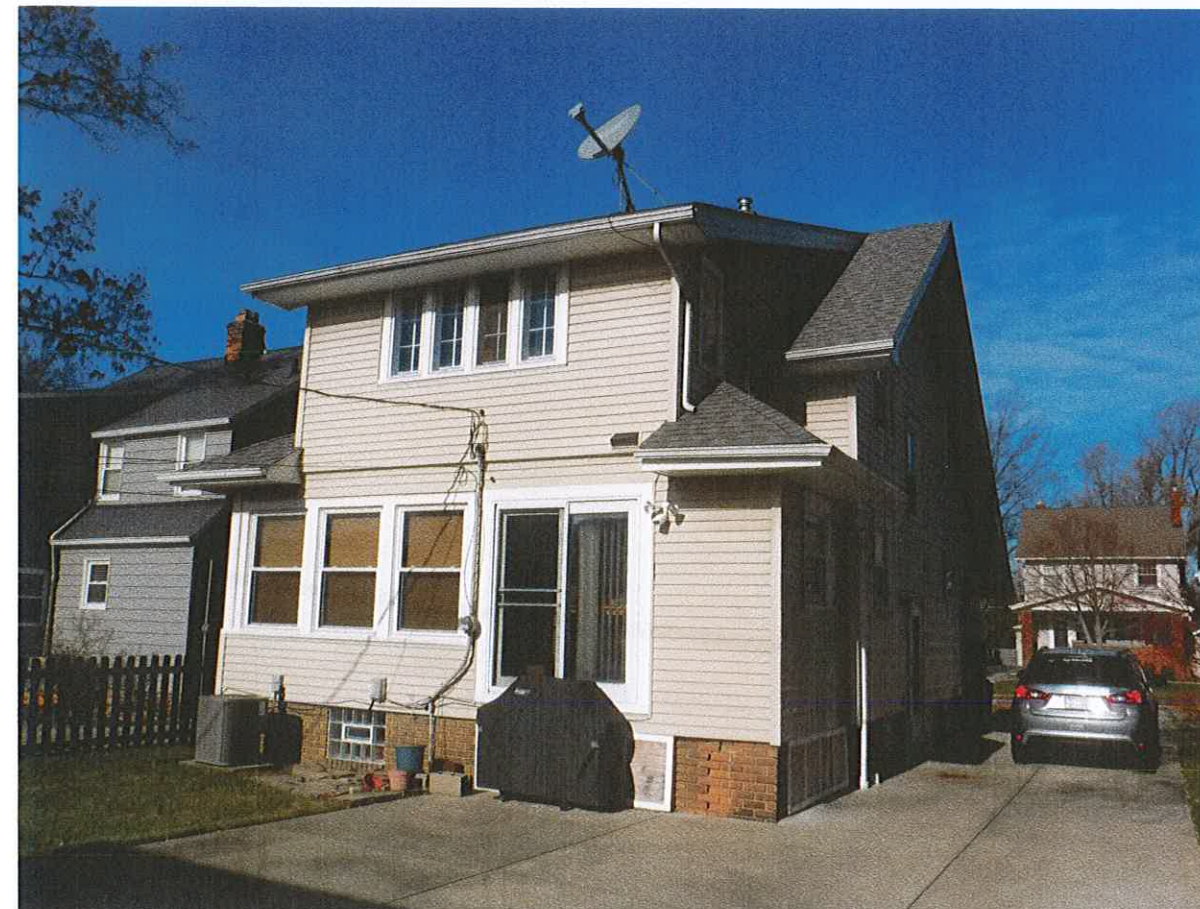
REAR OF EXISTING HOME VIEWING NORTHWEST
