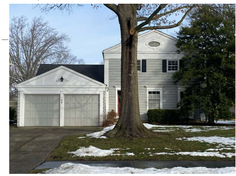
20760 - 2 DOORS TO THE WEST
