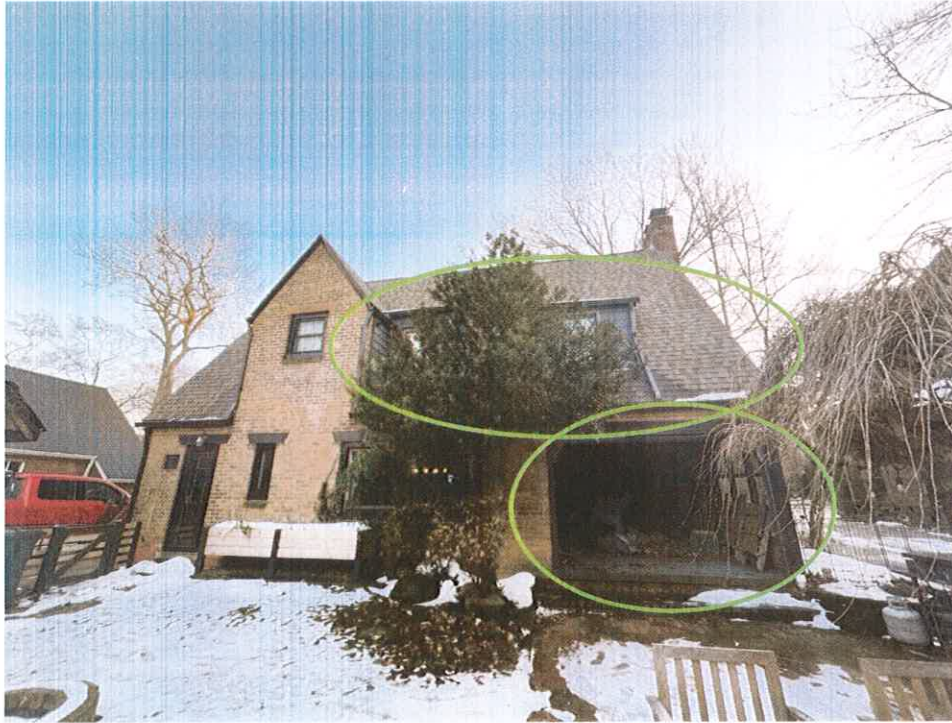
EXISTING REAR OF HOME (LOCATION OF PORCH ENCLOSURE ADDITION & DORMER ADDITION)
