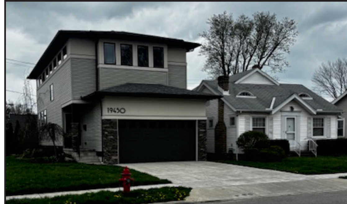
ADJACENT PROPERTY TO THE NORTH
