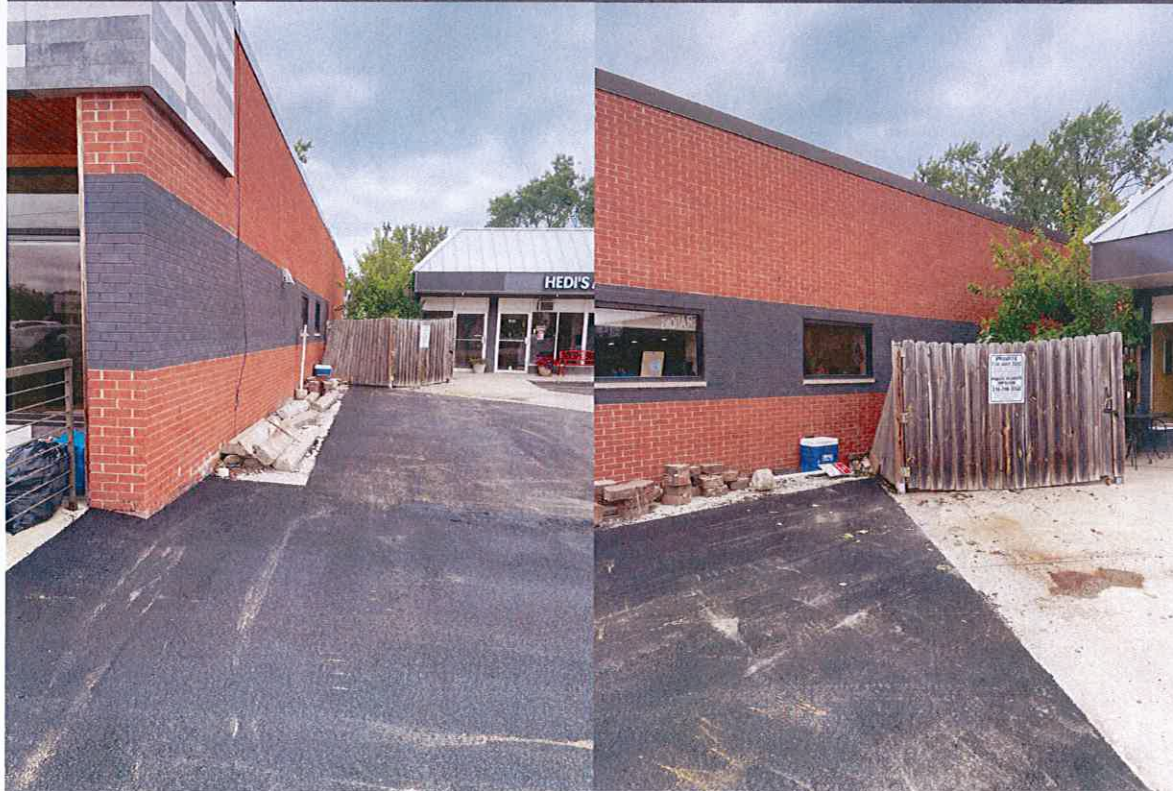
FRONT PARKING LOT
