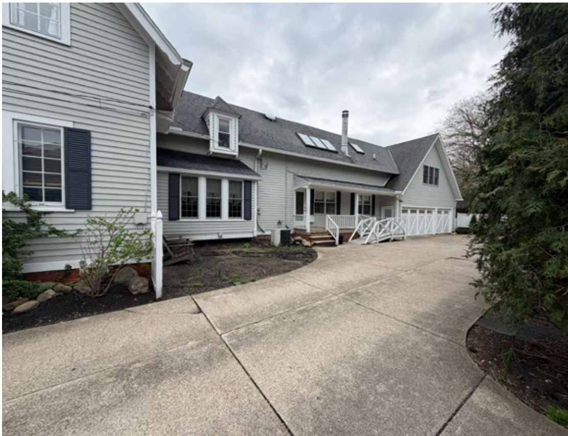
WEST SIDE OF HOUSE (LOOKING SOUTH)
