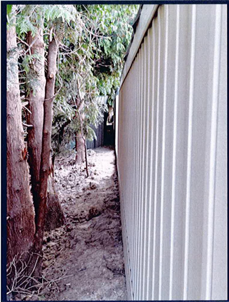
Residential side west facing
