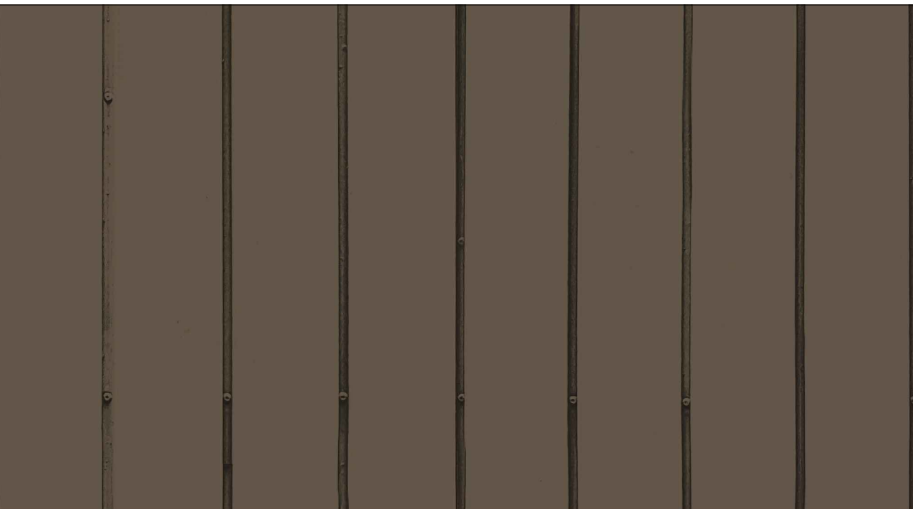
8 - Stained Vertical Cypress Siding to Match Trim Color of Existing House
