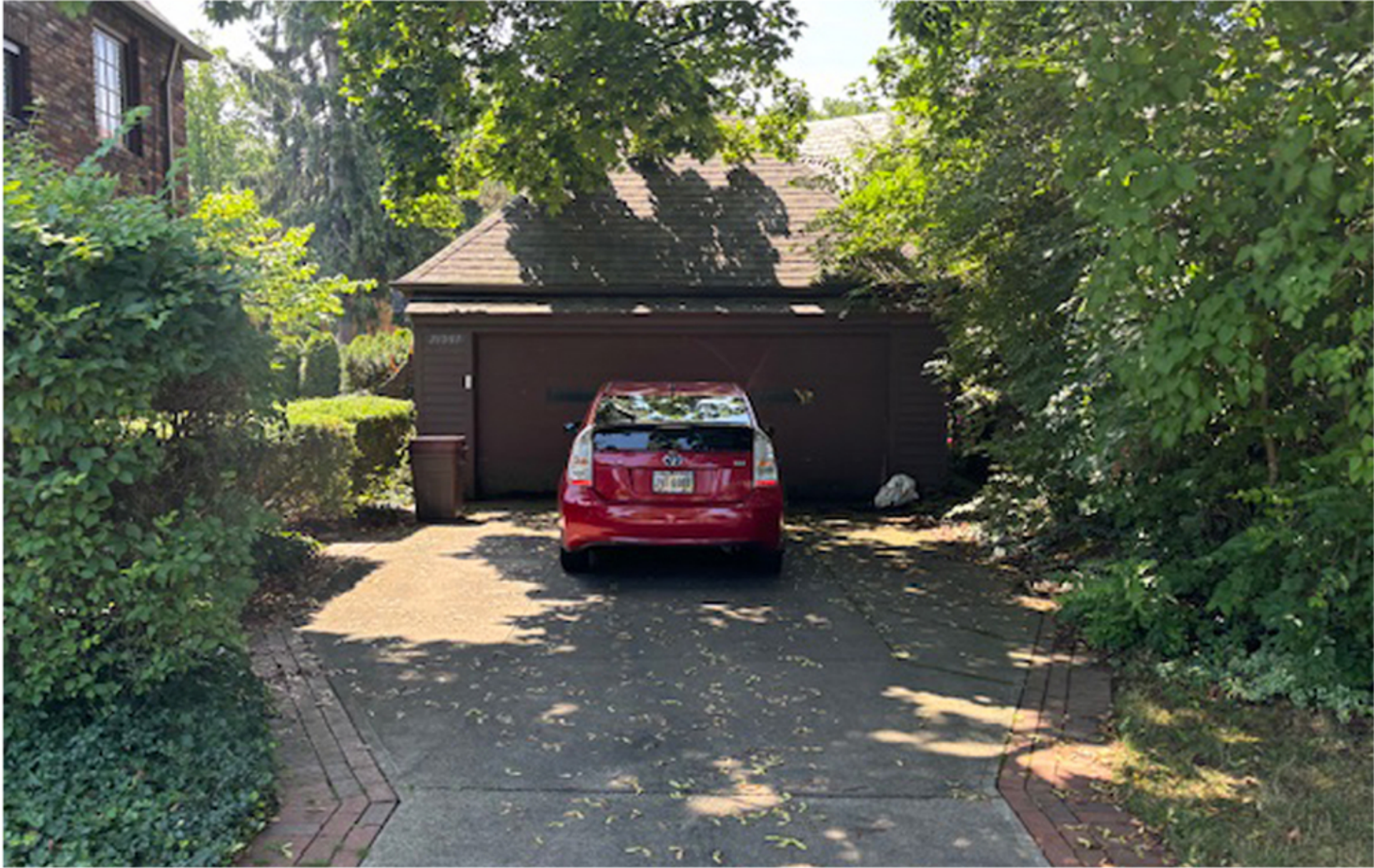
EXISTING NORTH ELEVATION (GARAGE)
