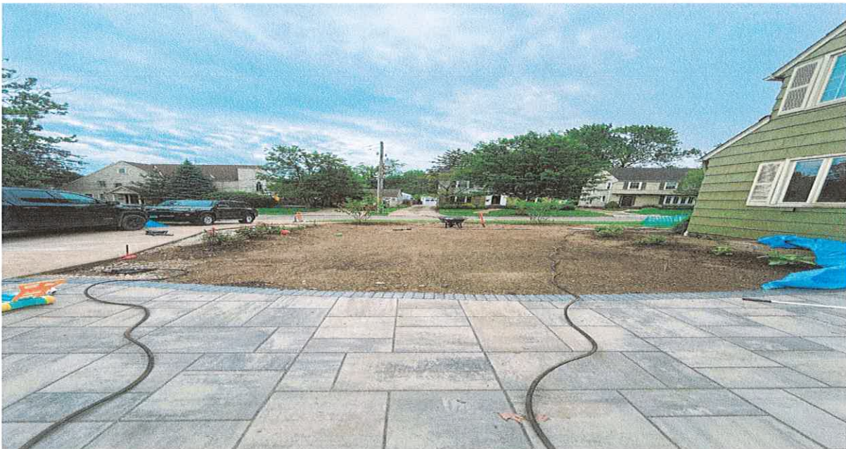
View from patio to front of yard facing Woodside. This would be the fenced in area allowing safe play for kids and dog
