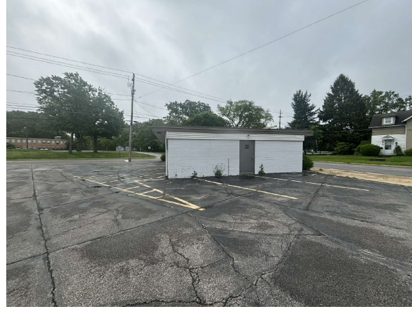
3 A102 NTS BUILDING A EXISTING EXTERIOR CONDITIONS
