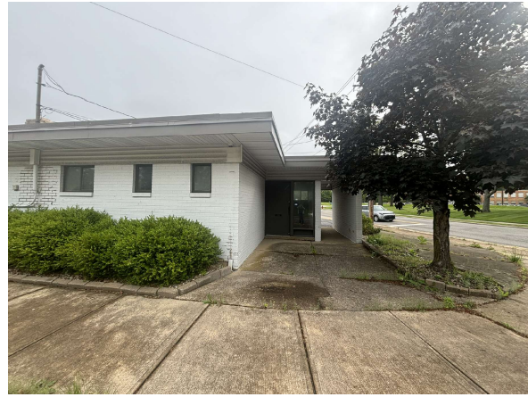
6 A102 NTS BUILDING A EXISTING EXTERIOR CONDITIONS
