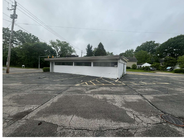
2 A102 NTS BUILDING A EXISTING EXTERIOR CONDITIONS
