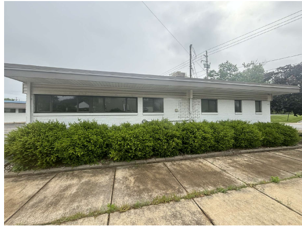
5 A102 NTS BUILDING A EXISTING EXTERIOR CONDITIONS
