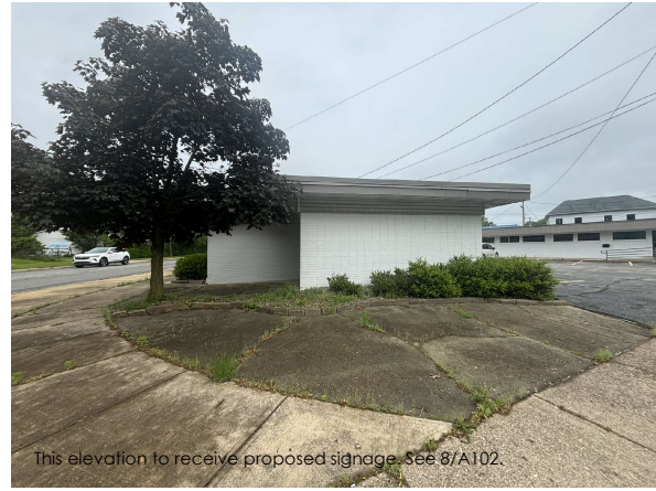
7 A102 NTS BUILDING A EXISTING EXTERIOR CONDITIONS
