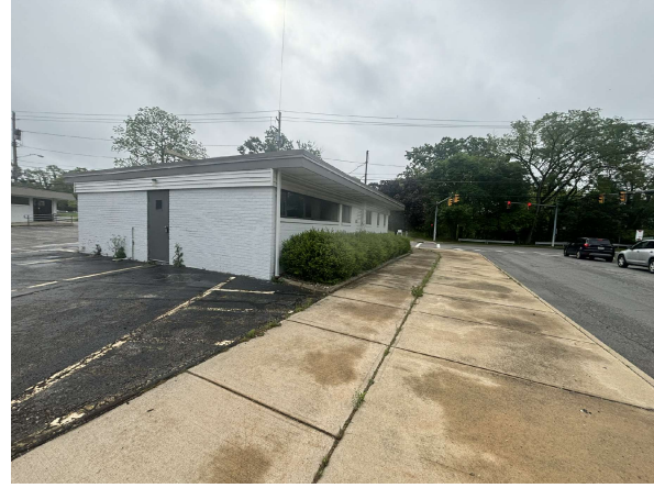
4 A102 NTS BUILDING A EXISTING EXTERIOR CONDITIONS
