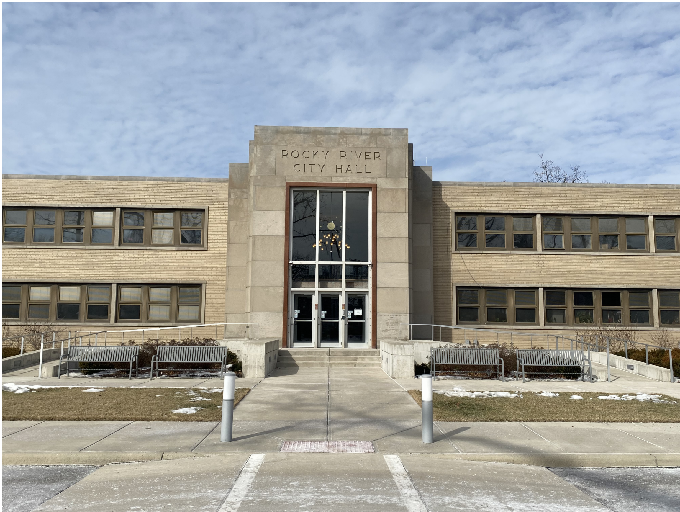
EXISTING CITY HALL
