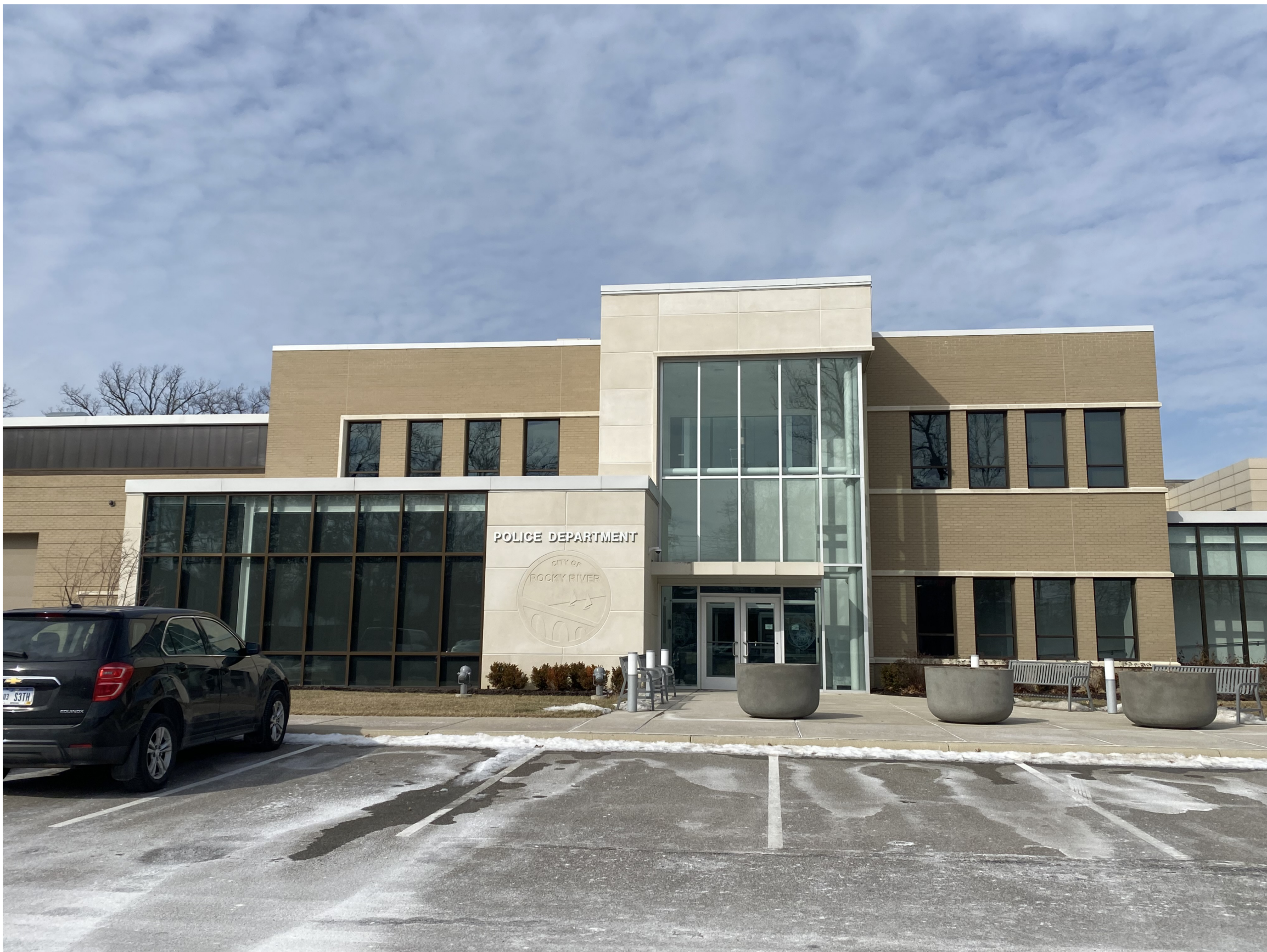
EXISTING POLICE STATION
