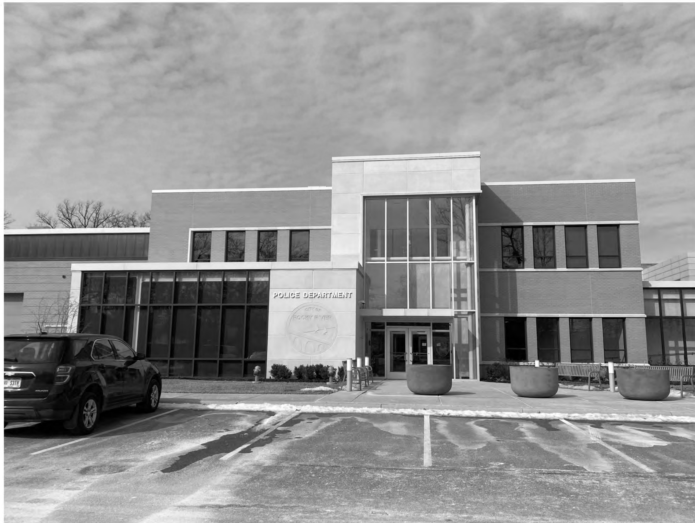
EXISTING POLICE STATION
