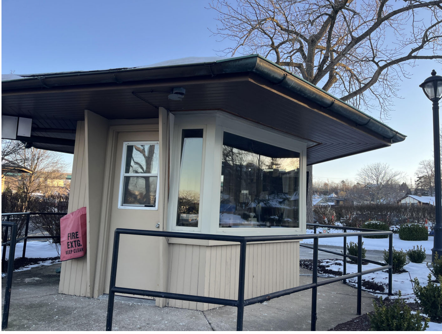
EXISTING GATEHOUSE WEST
