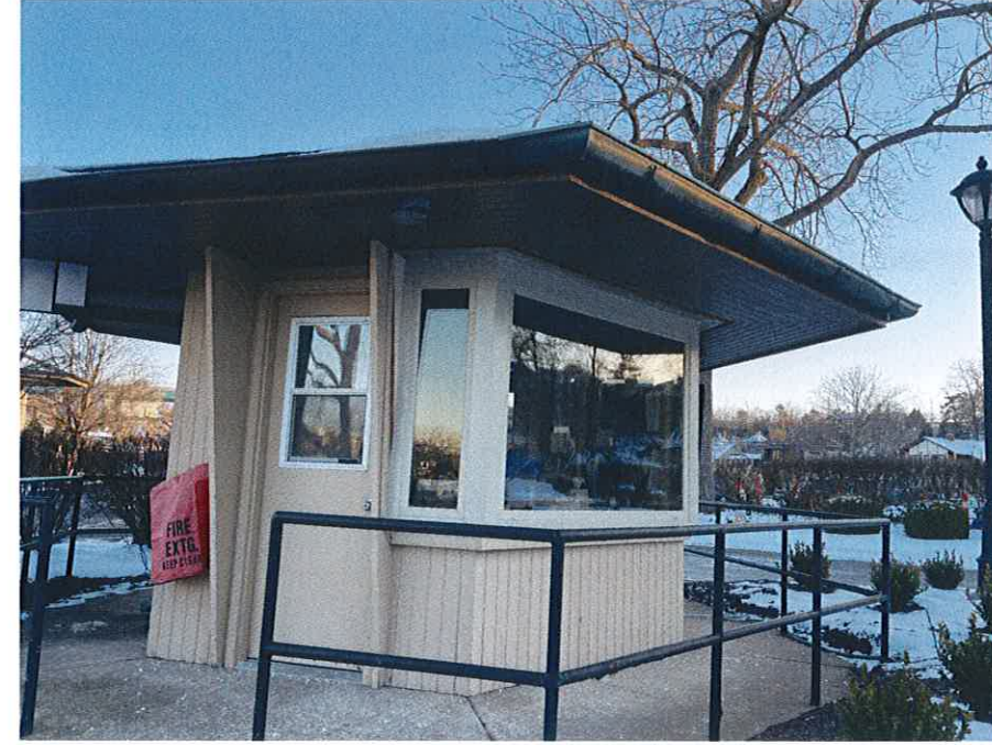
EXISTING GATEHOUSE WEST
