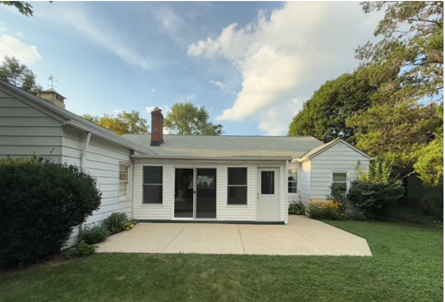
Hecker Residence rear elevation
