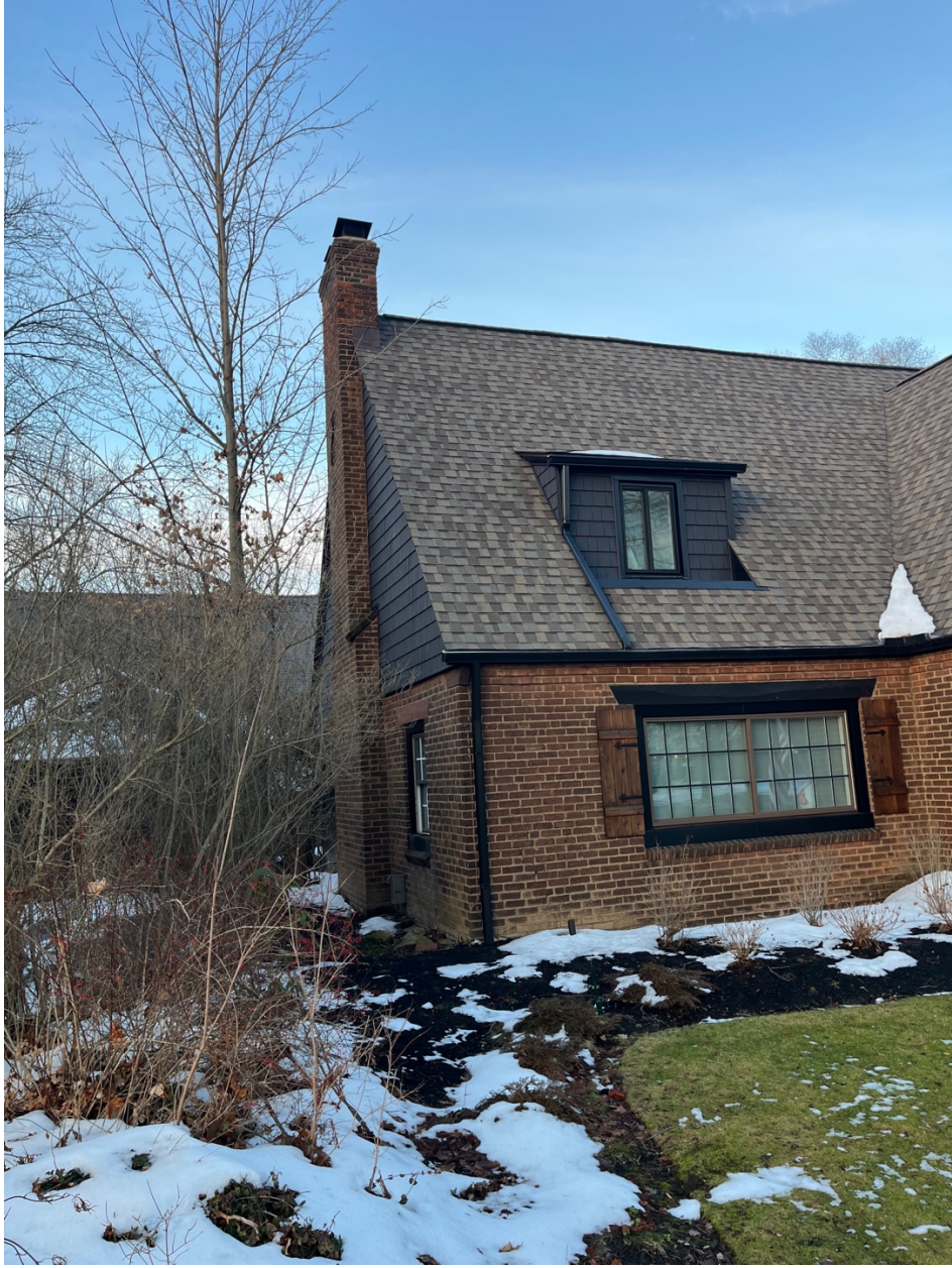
EXISTING LEFT SIDE OF HOME (FROM FRONT LEFT CORNER)
