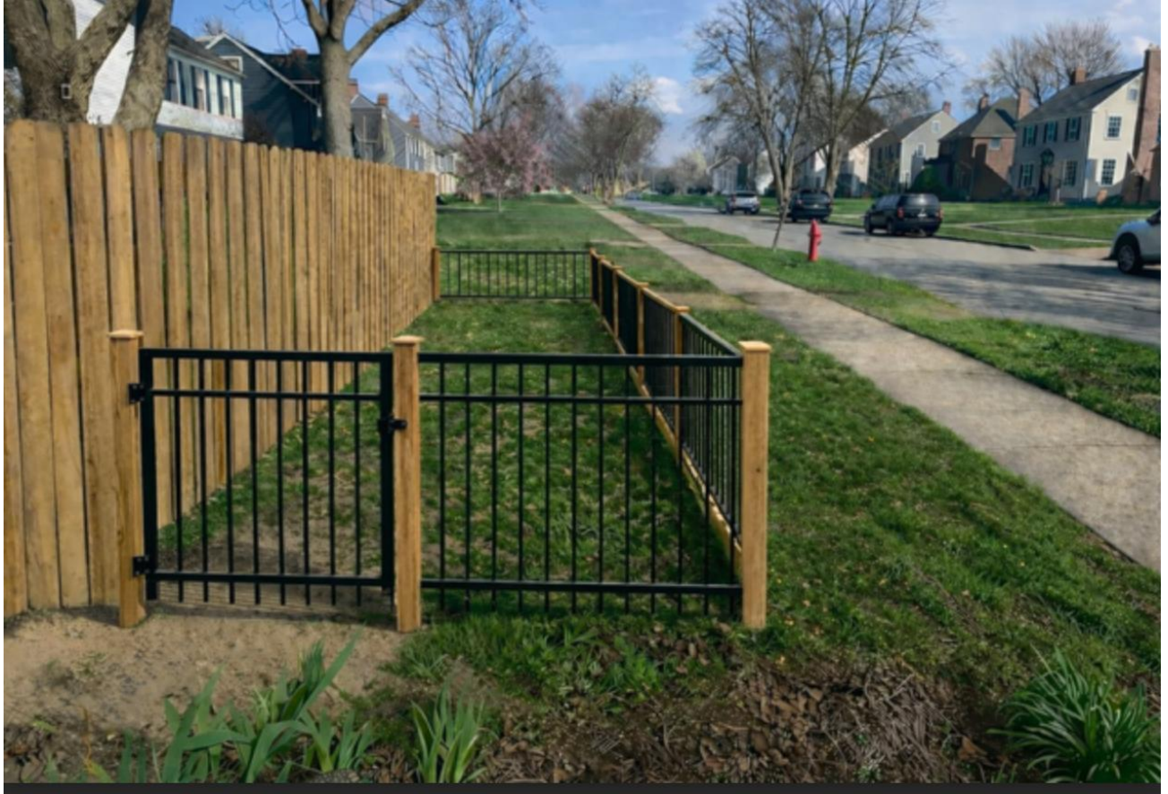
42-inch ornamental fence
