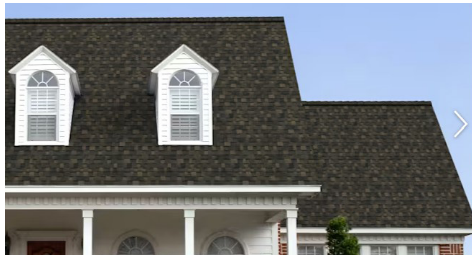
Owens Corning - Black Sable Roof
