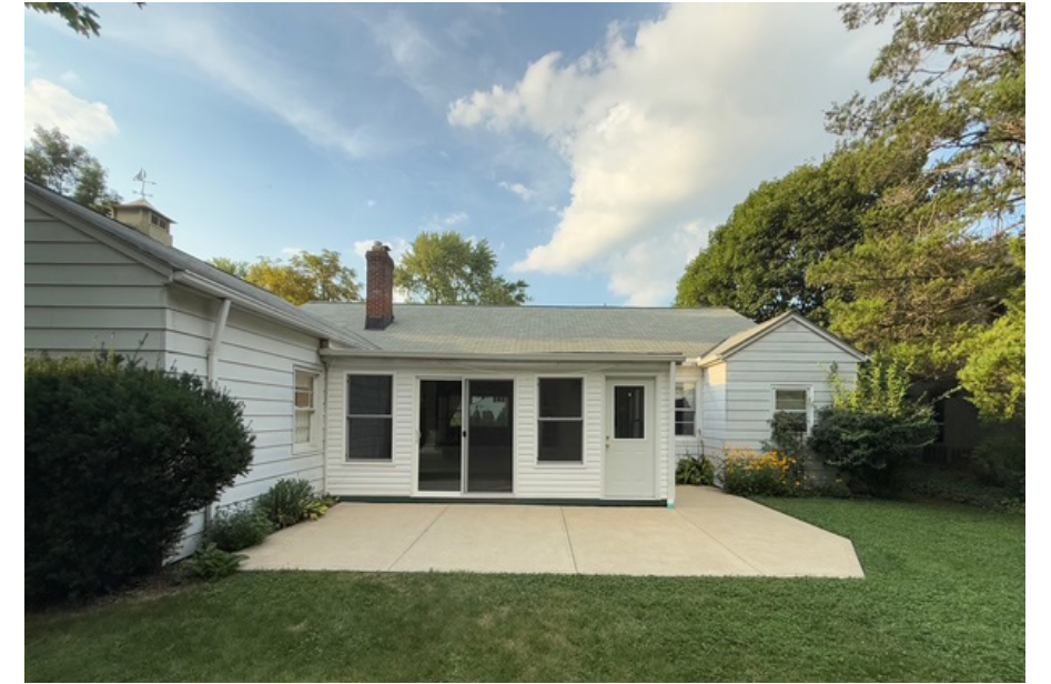
Hecker Residence rear elevation
