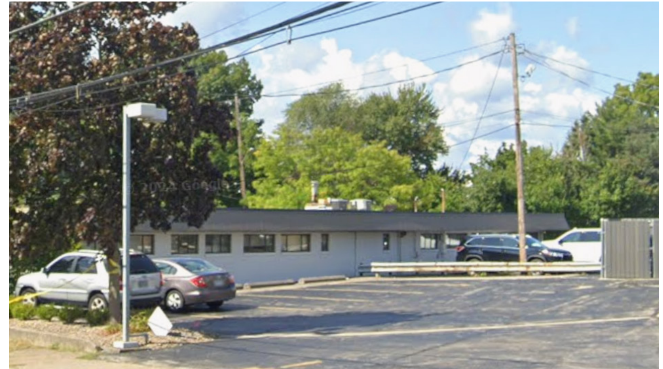
VIEW FROM WOOSTER RD (NORTH ELEVATION)
