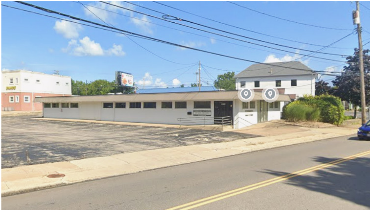
VIEW FROM WOOSTER RD (SOUTH ELEVATION)
