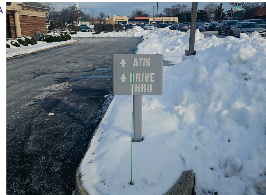
Existing 18" x 21-3/4" directional sign to be removed & replaced
