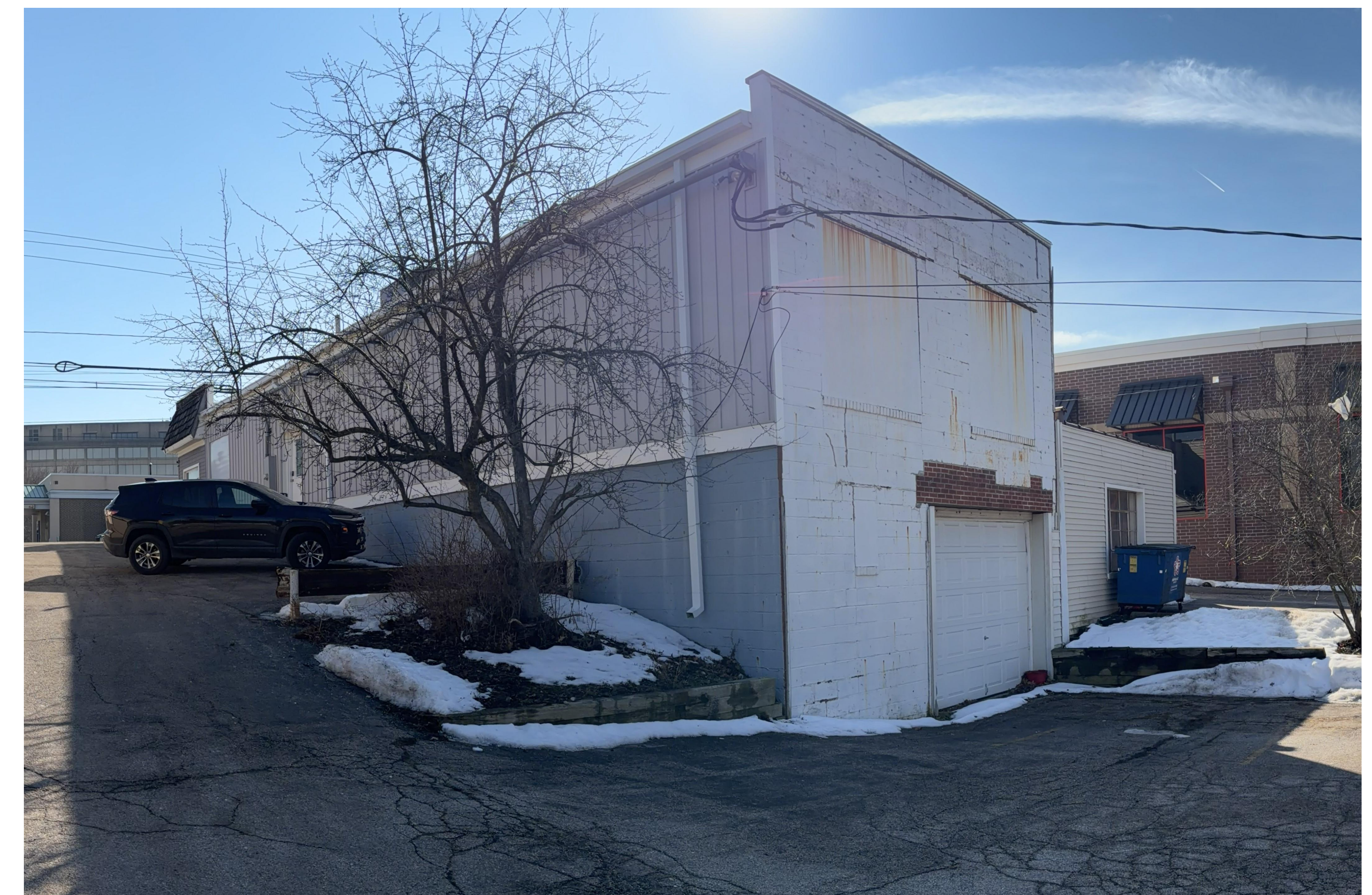
20350 & 20370 BUILDING NORTH FACADE
