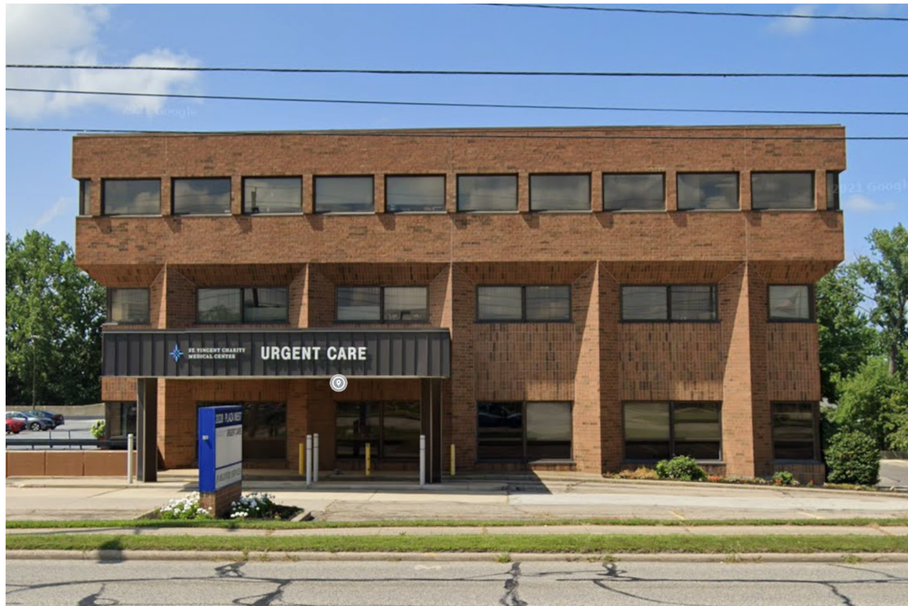
2020 BUILDING SOUTH FACADE
