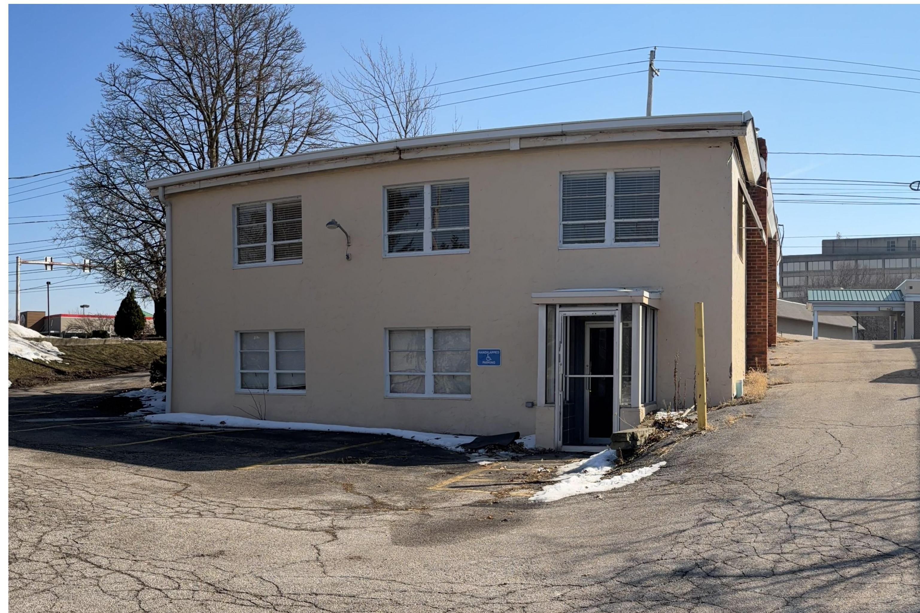
20340 BUILDING NORTH FACADE (TO BE DEMOLISHED)
