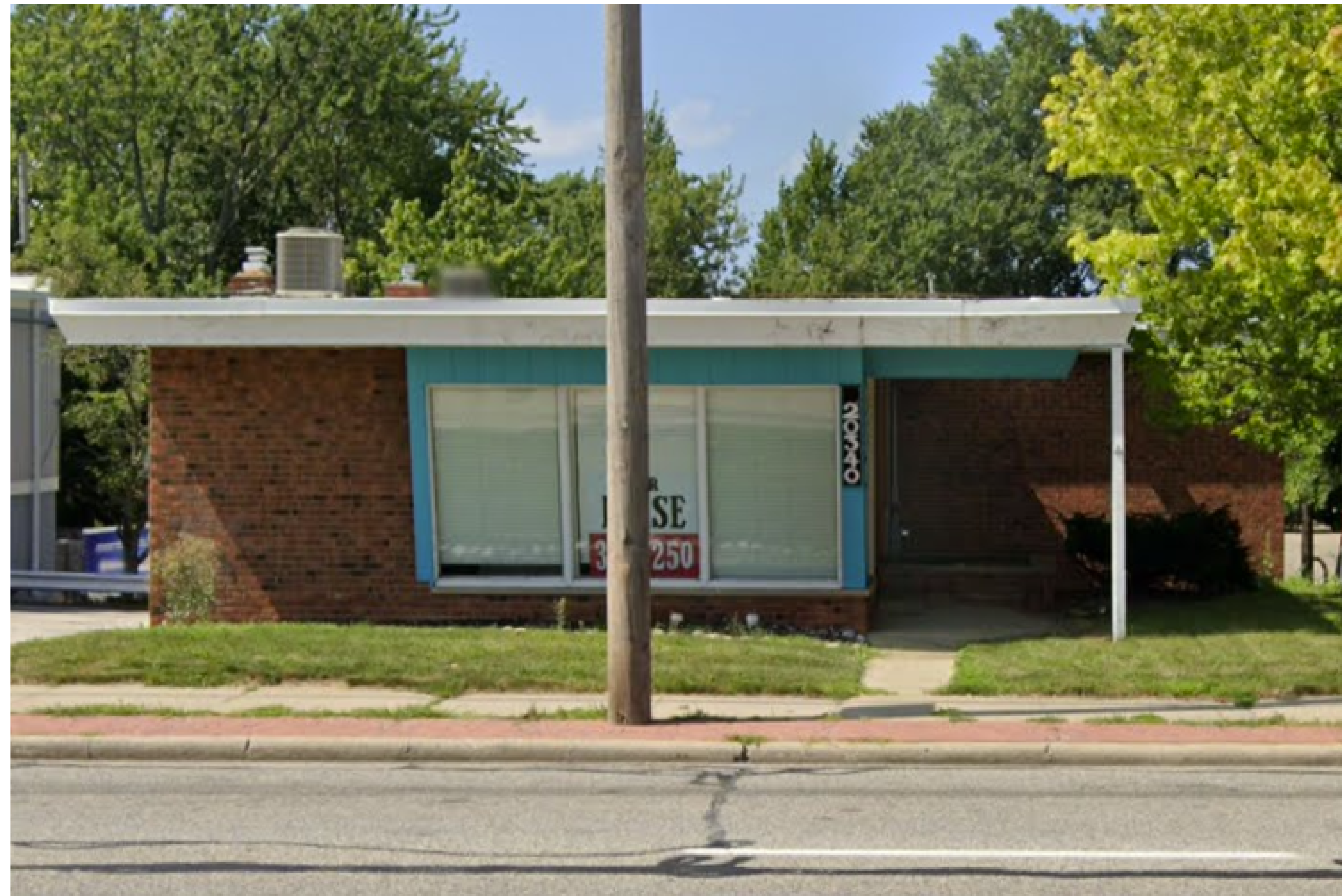
20340 BUILDING SOUTH FACADE (TO BE DEMOLISHED)
