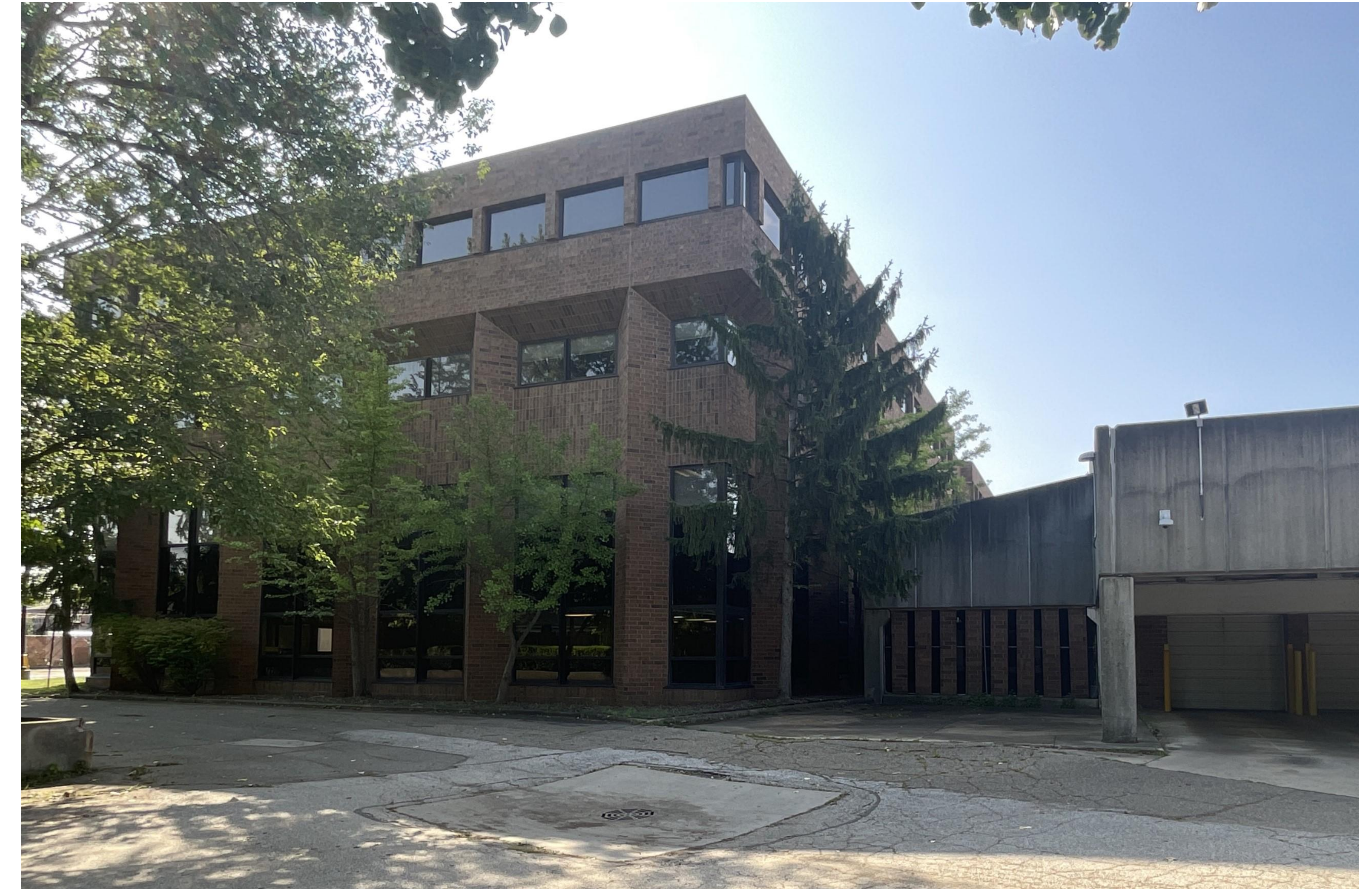
2020 BUILDING NORTH FACADE
