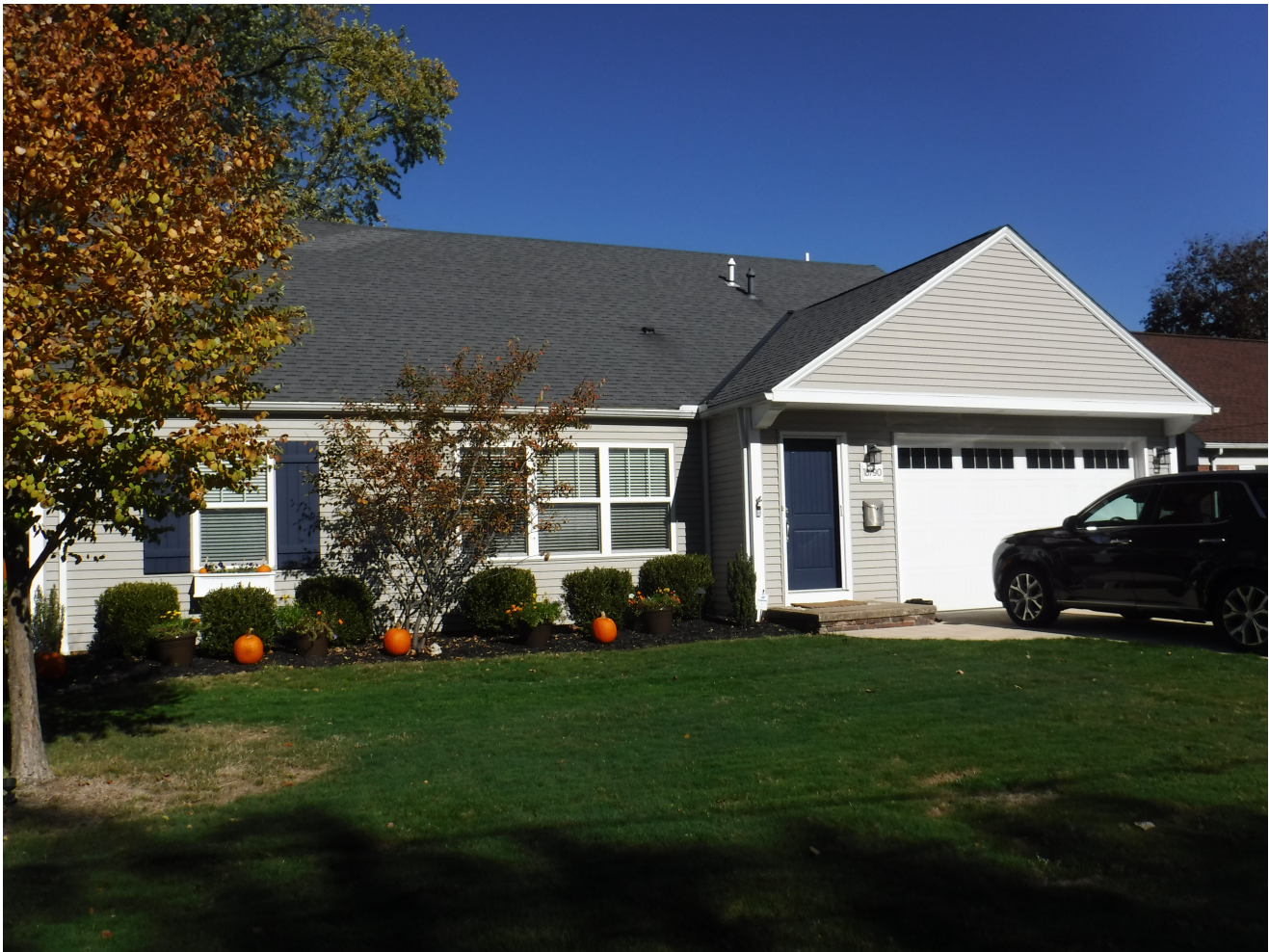
EXISTING CONDITIONS PHOTO VIEWING NORTHEAST
