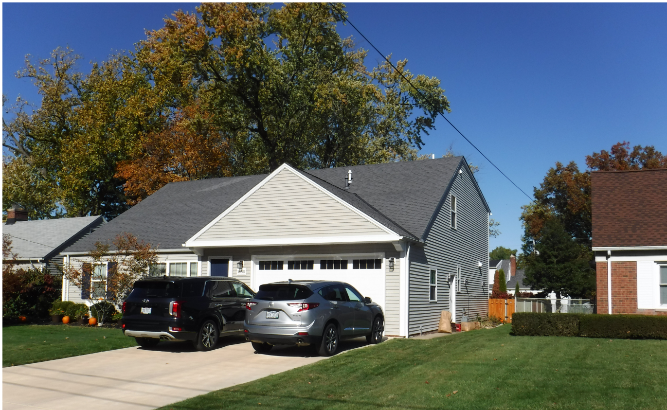
EXISTING CONDITIONS PHOTO VIEWING NORTHWEST
