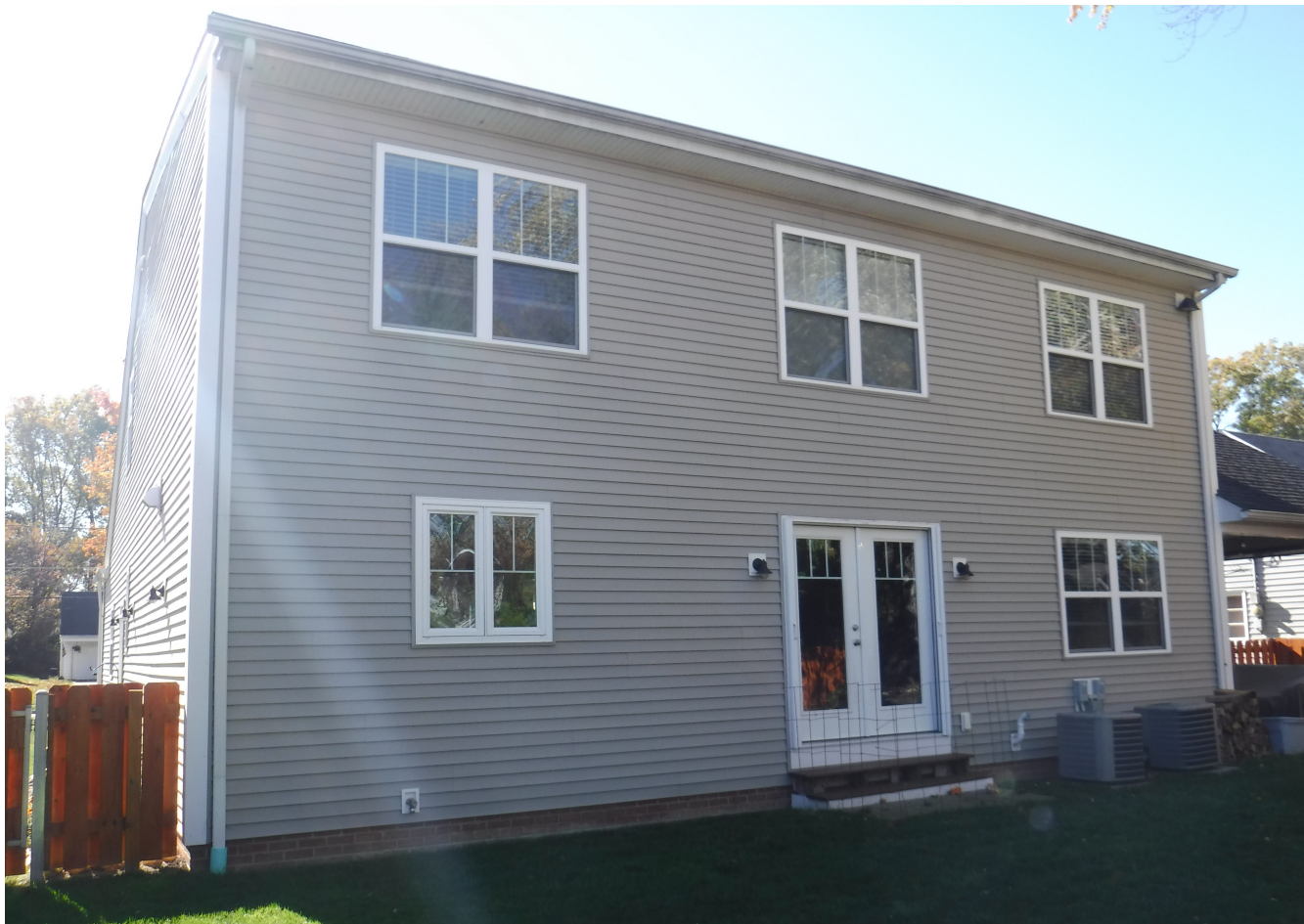
EXISTING CONDITIONS PHOTO VIEWING SOUTHWEST
