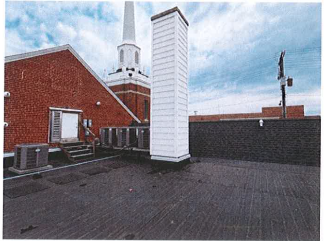
Proposed siding repairs using white clapboard vinyl siding consistent with existing colors already on the building.
