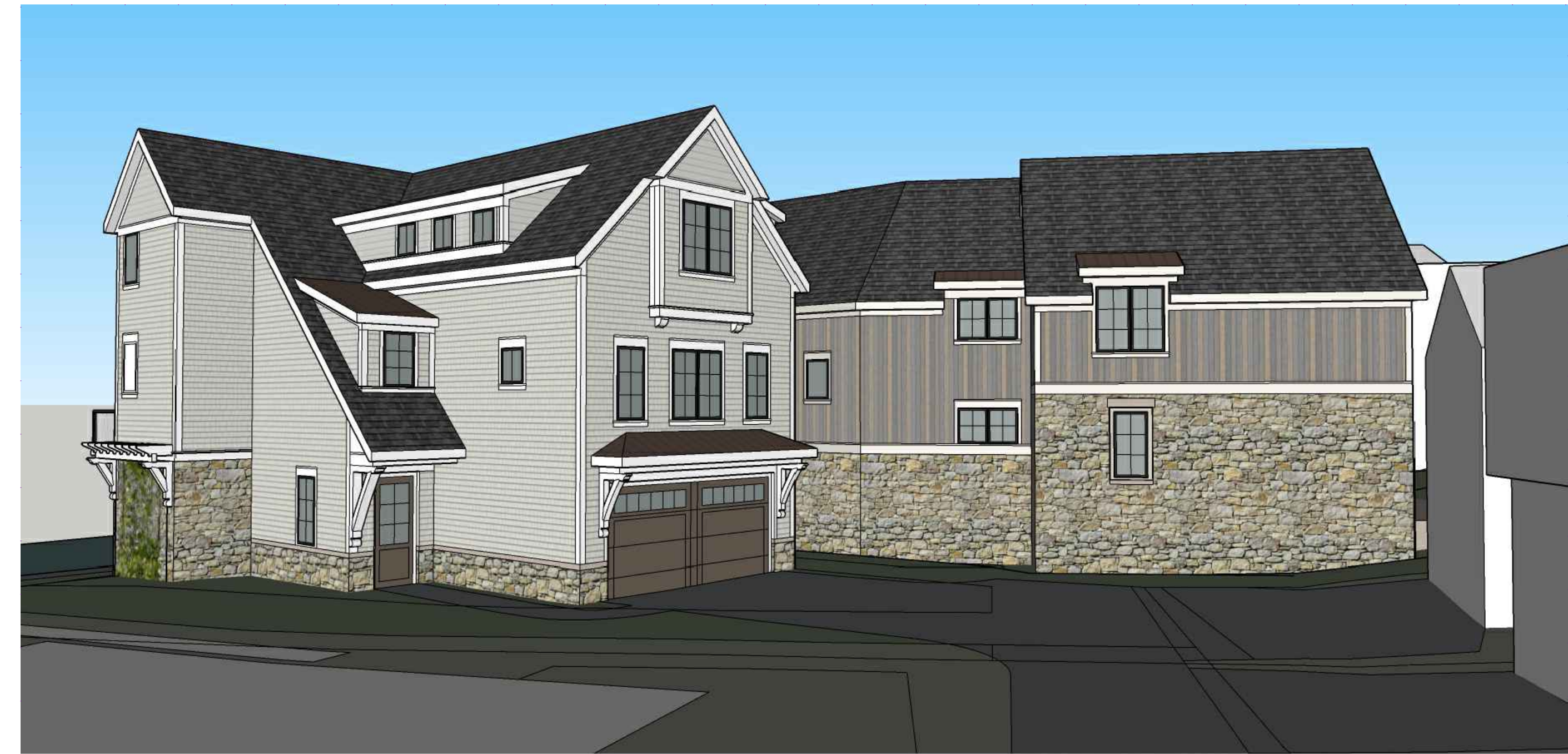
South Island Drive - Looking SE
