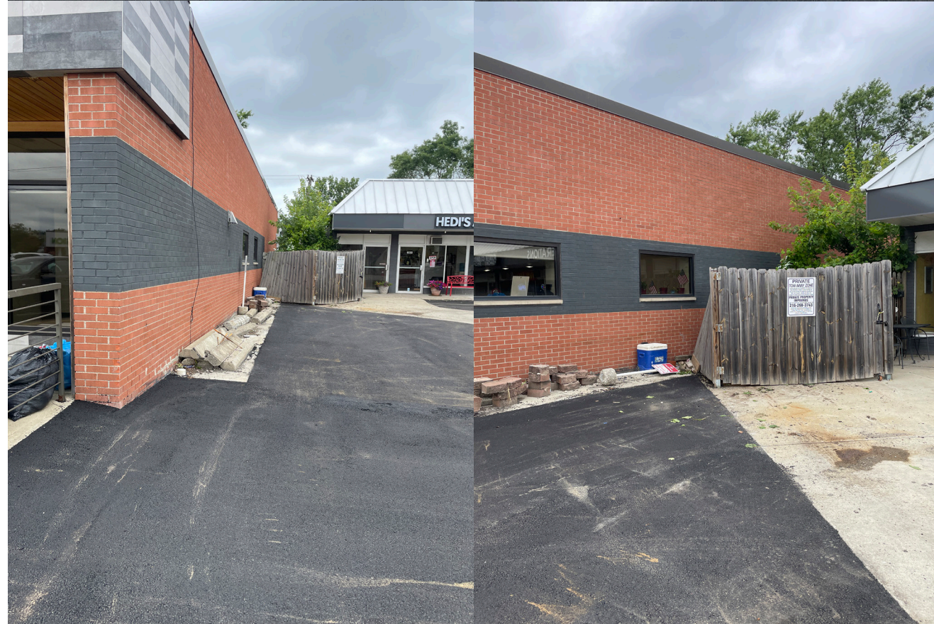
FRONT PARKING LOT
