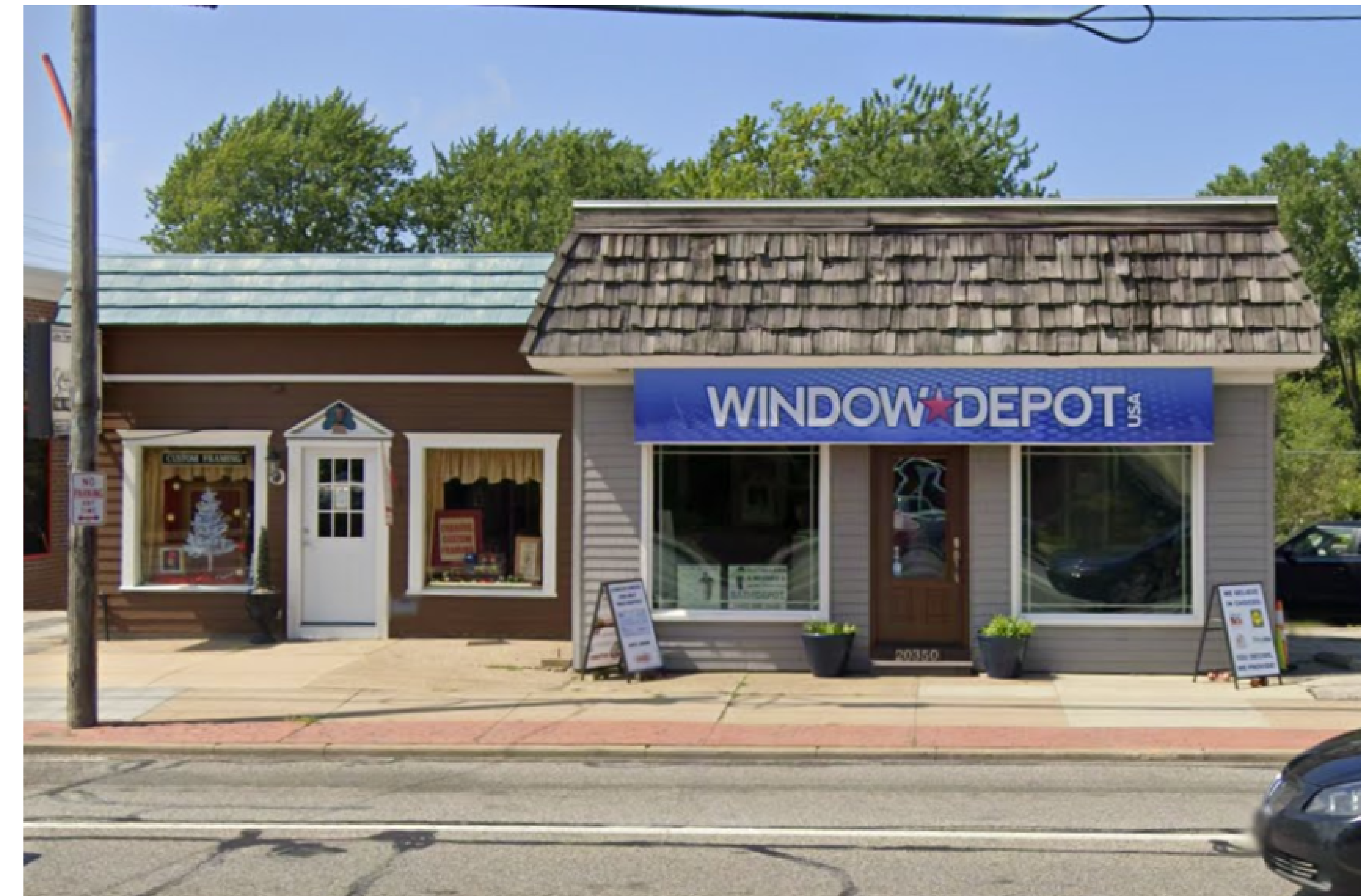
20350 & 20370 BUILDING SOUTH FACADE
