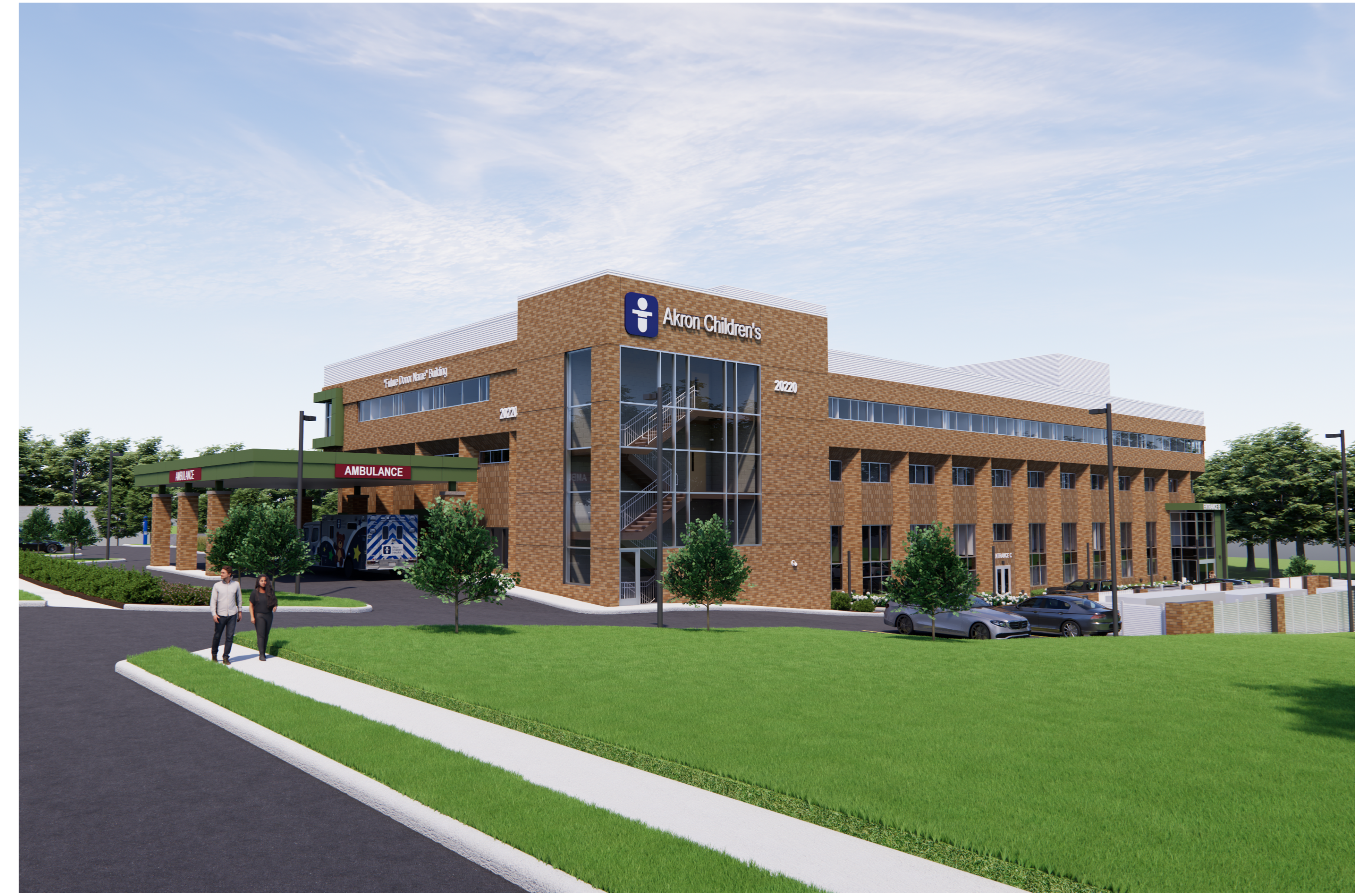
STREET VIEW EAST FACADE
