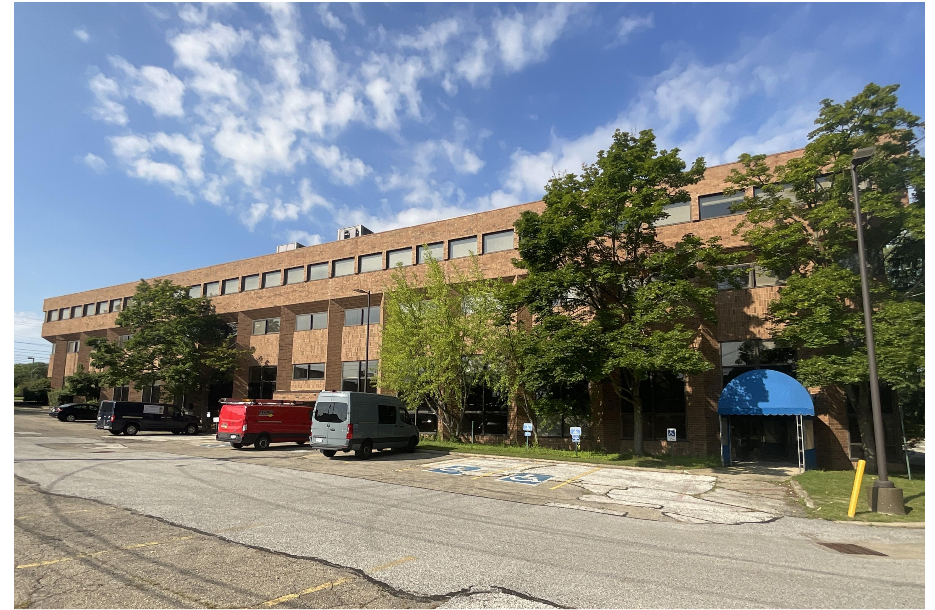
2020 BUILDING EAST FACADE
