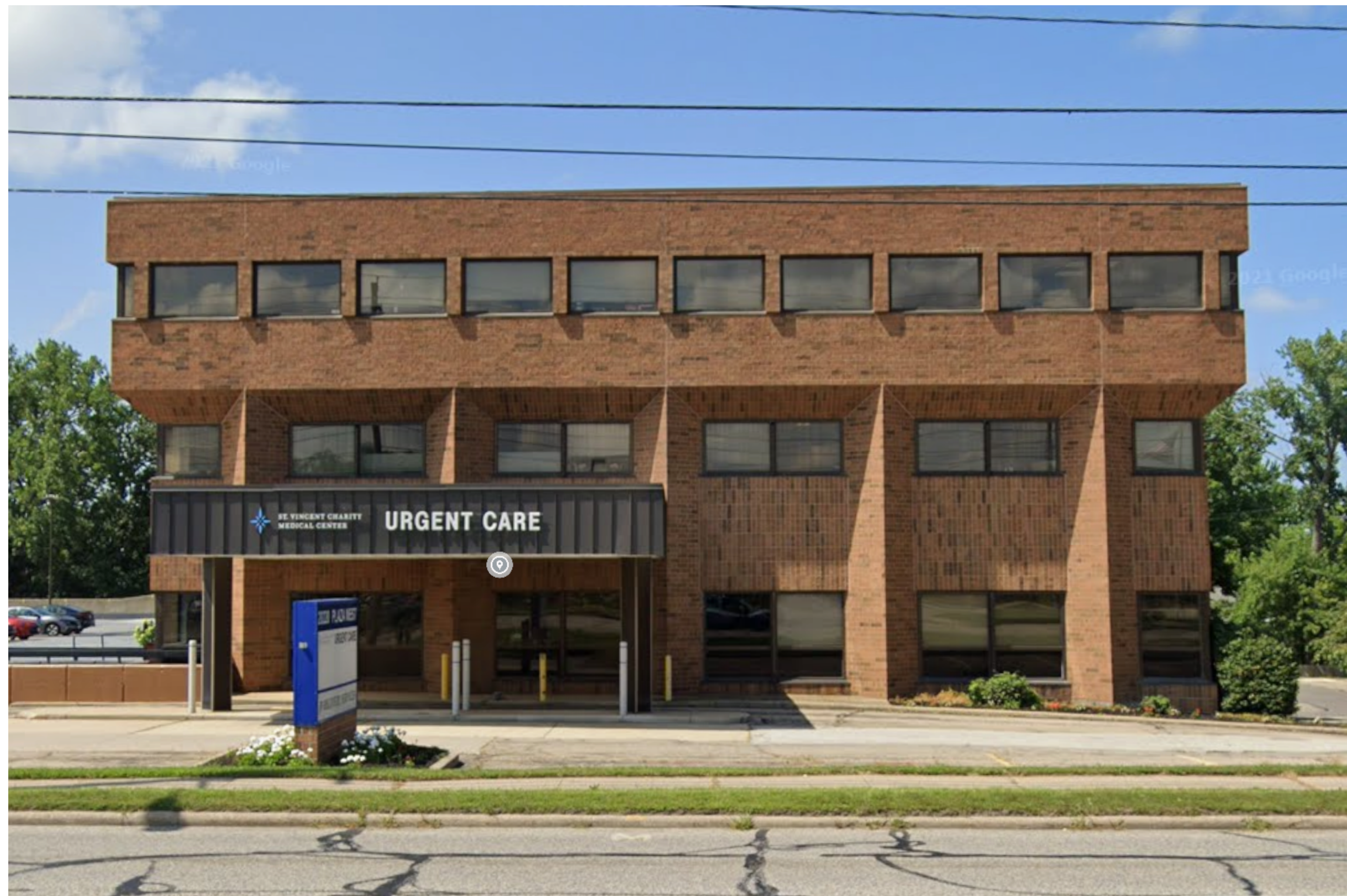
2020 BUILDING SOUTH FACADE
