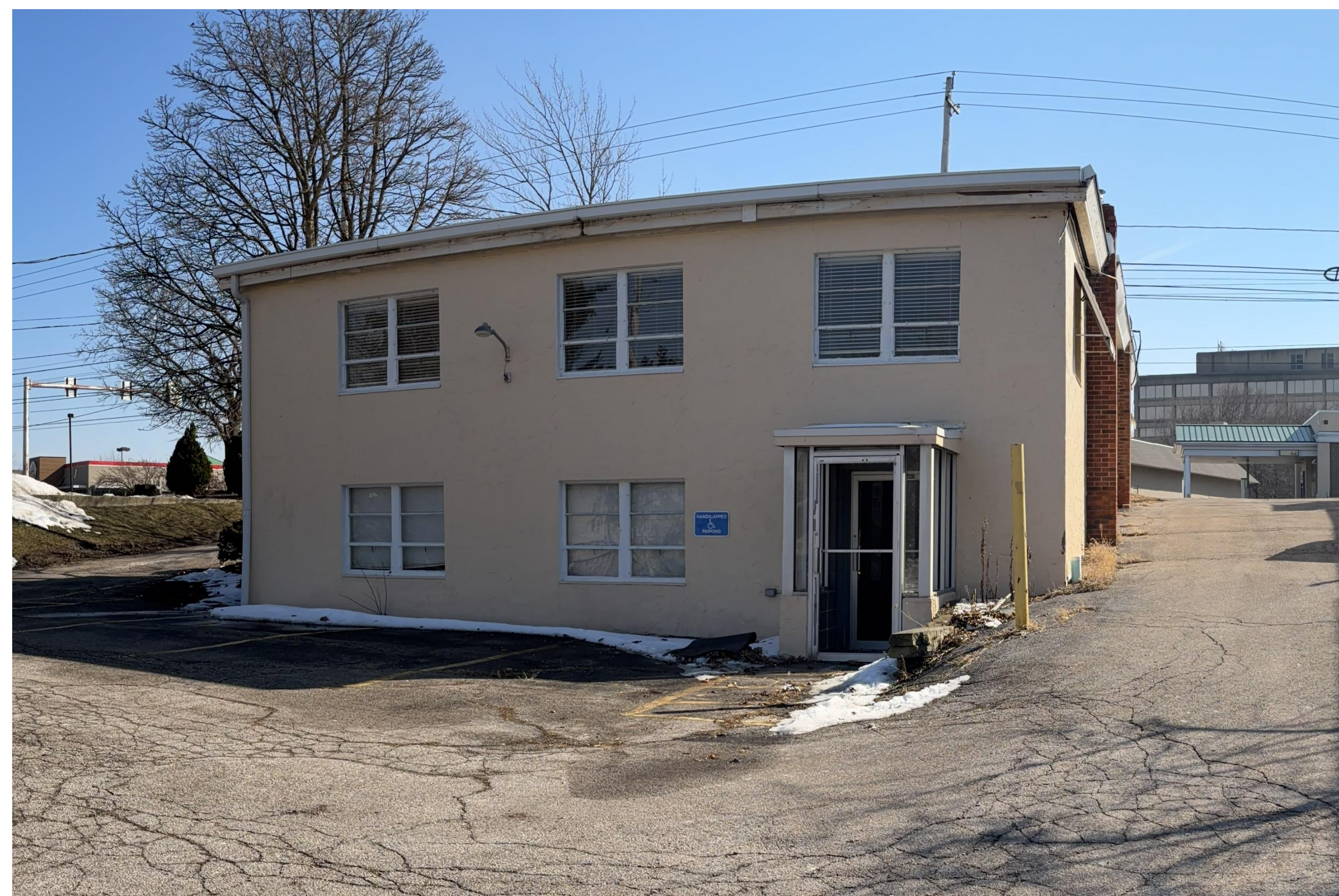
20340 BUILDING NORTH FACADE (TO BE DEMOLISHED)
