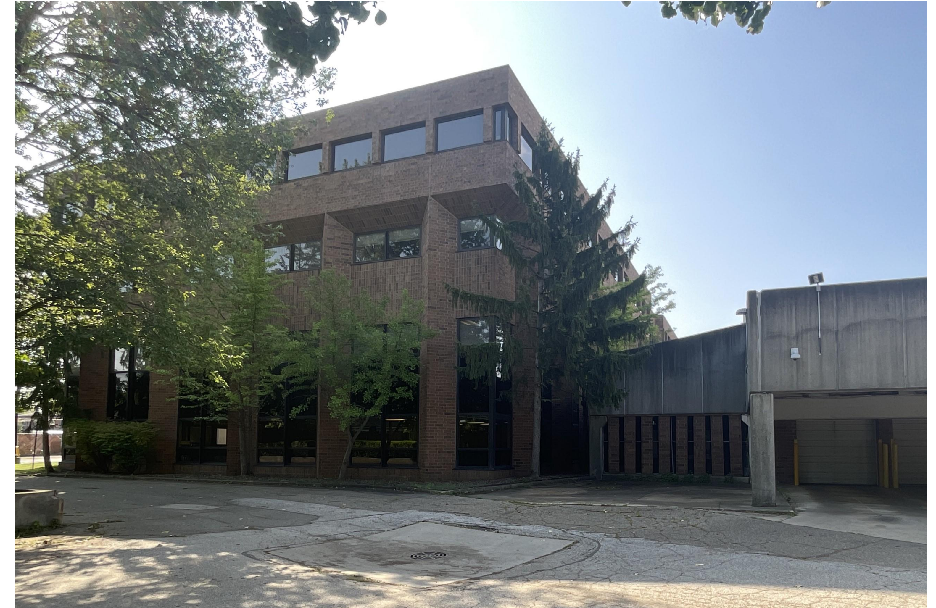
2020 BUILDING NORTH FACADE
