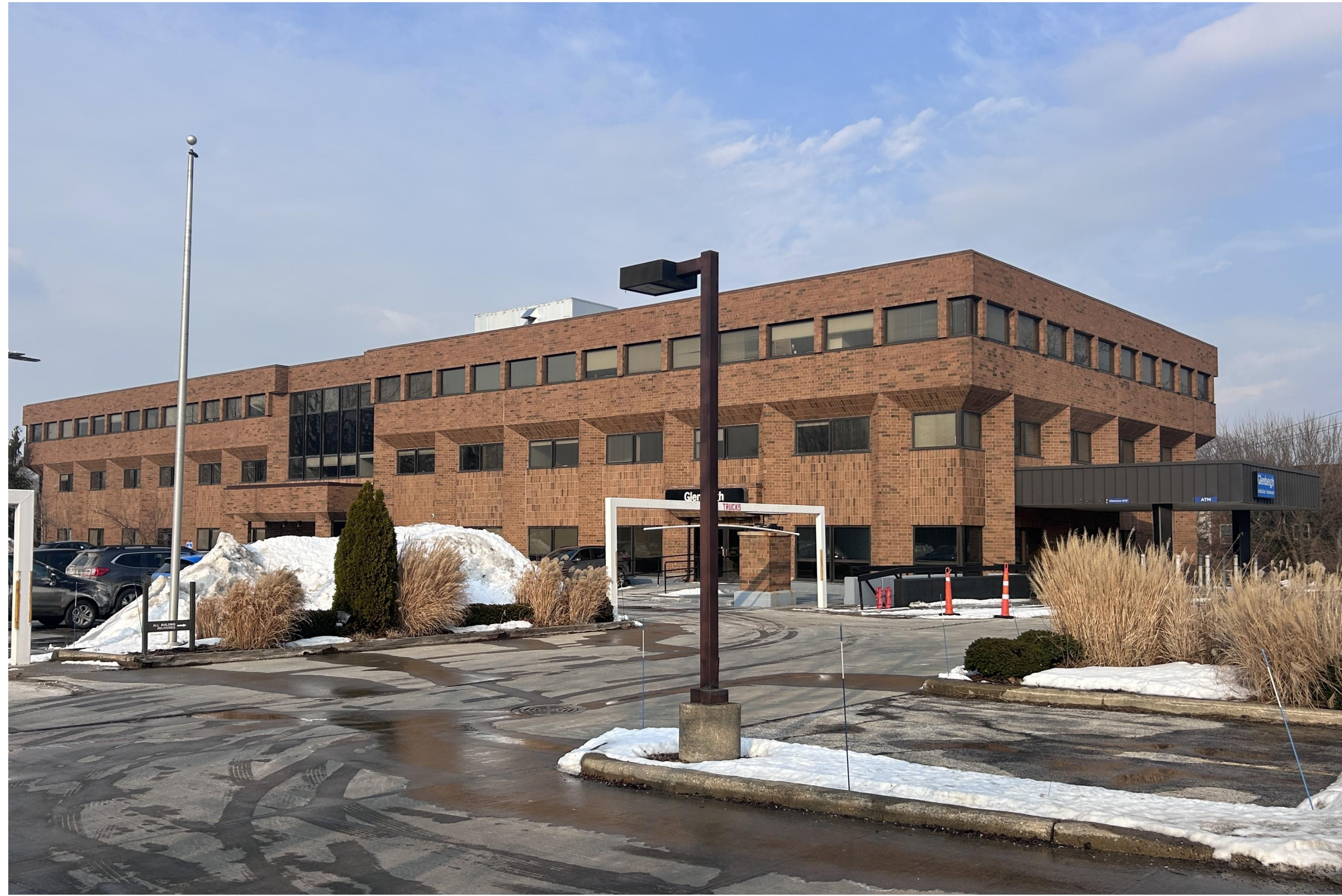
2020 BUILDING WEST FACADE
