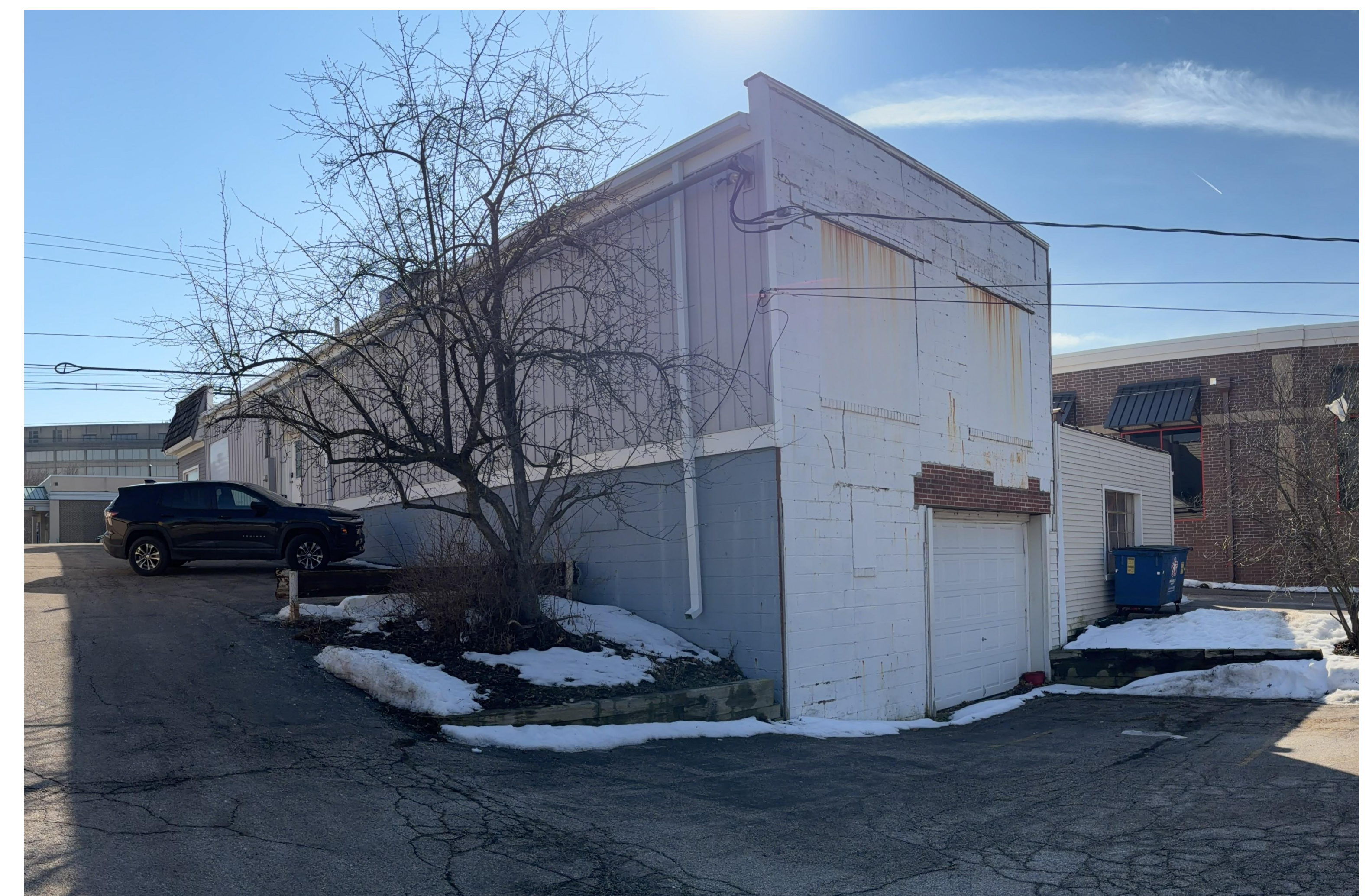
20350 & 20370 BUILDING NORTH FACADE
