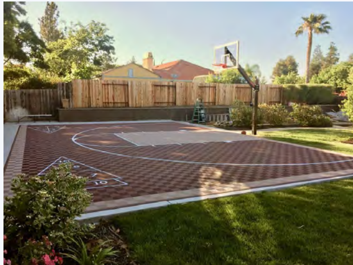
Representative example: poured concrete base finished with interlocking multi-sport tiles and portable hoop.
