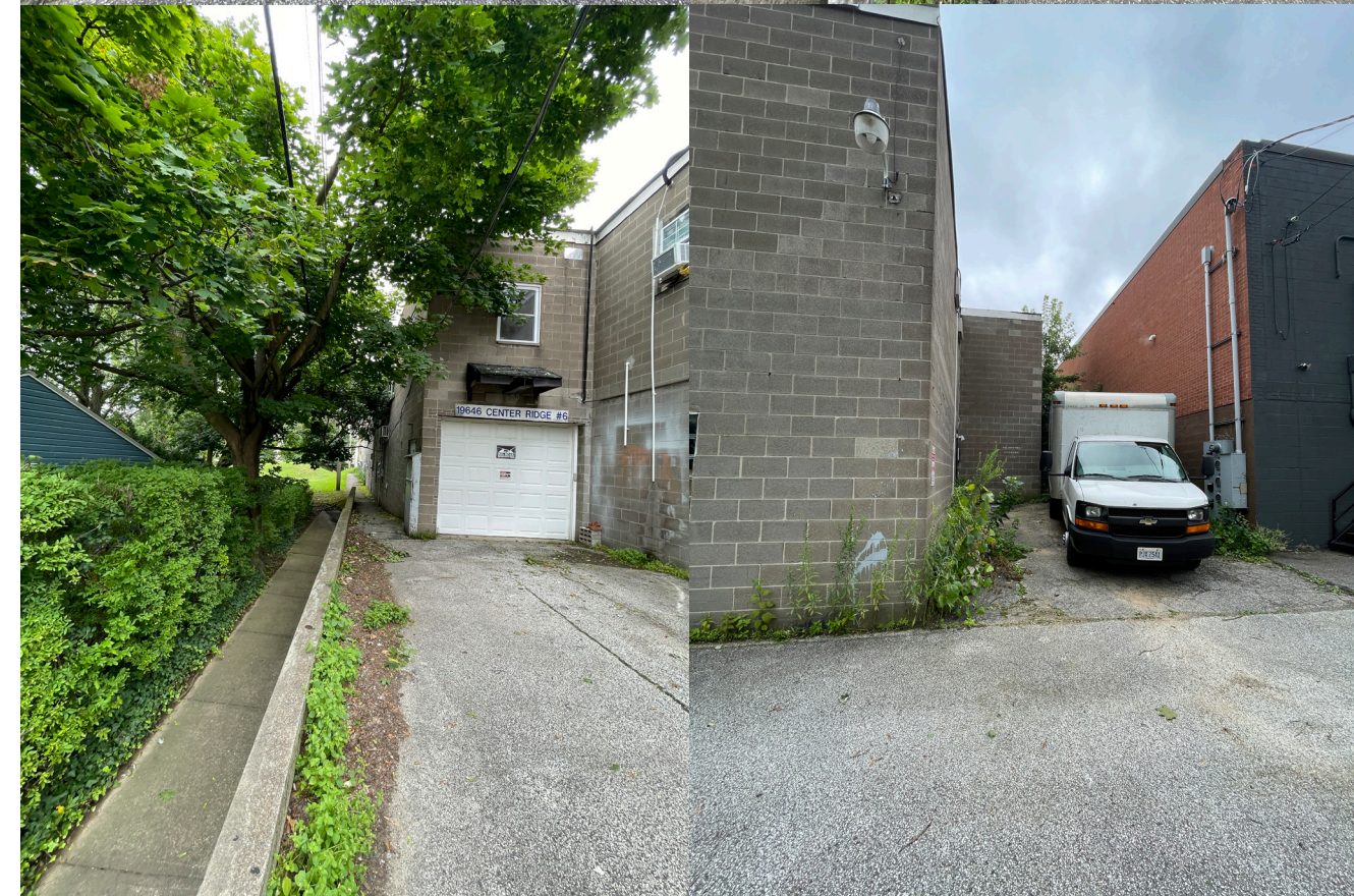
REAR PARKING/GARAGE ENTRANCE
