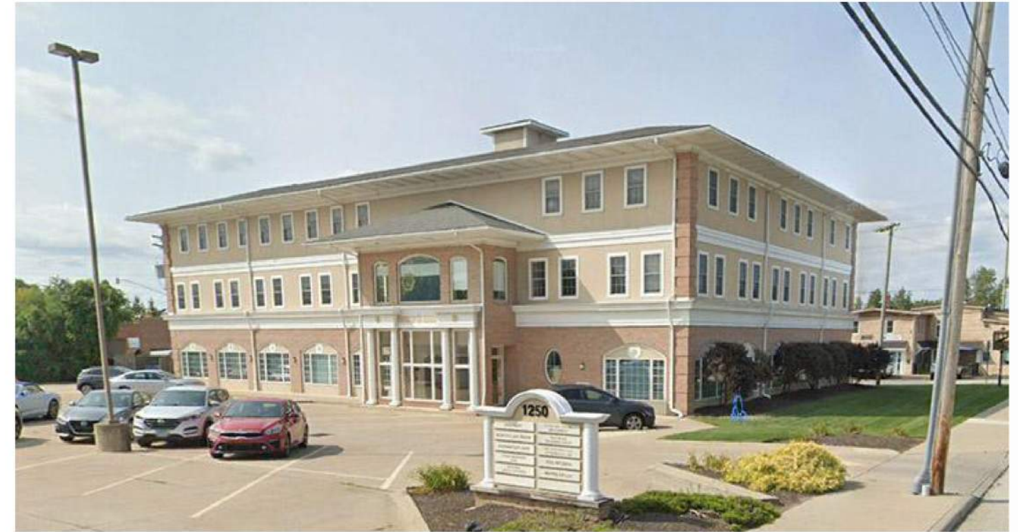
Looking North at 1250 Linda St.
