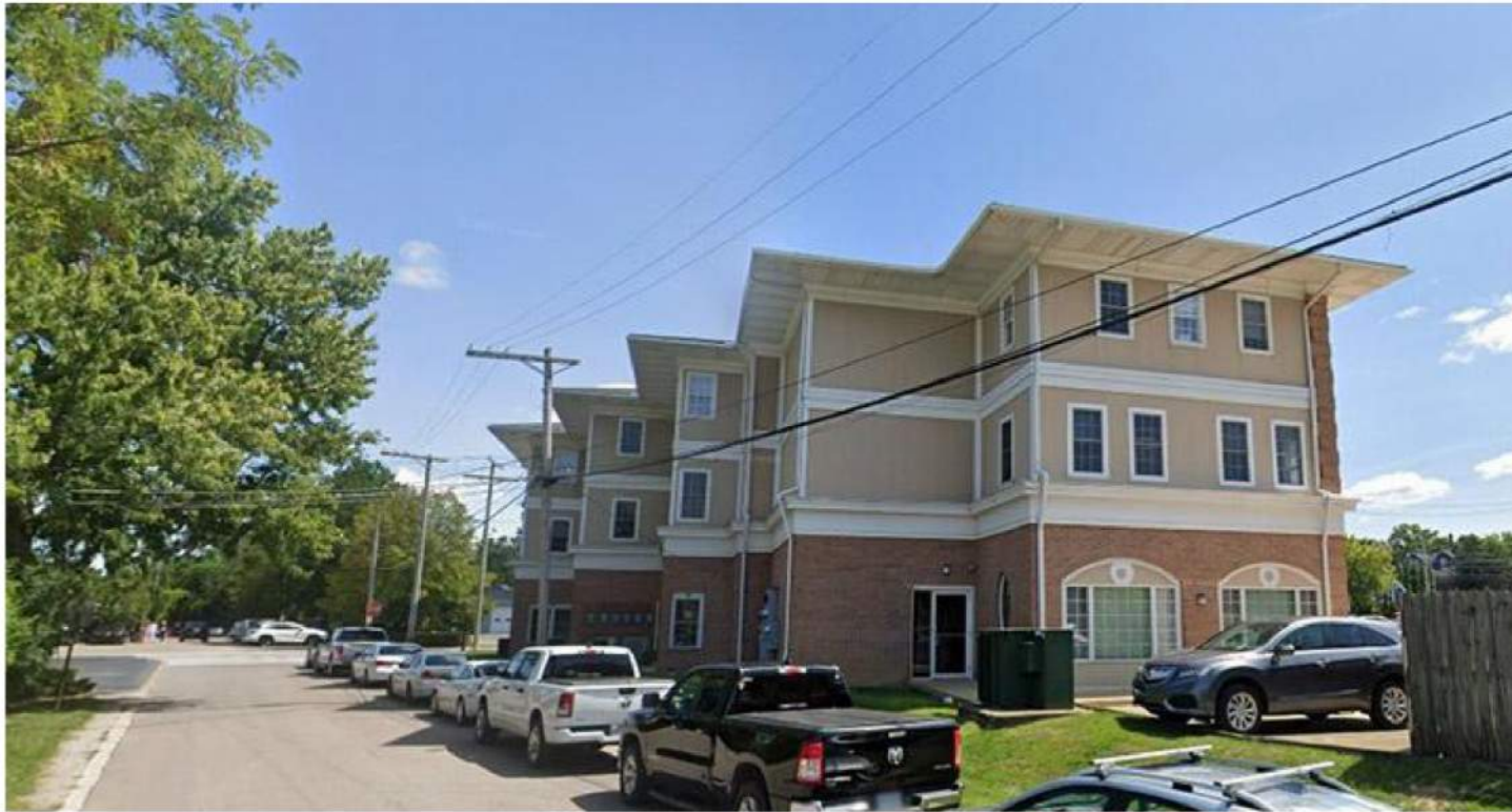
Looking East at 1250 Linda from Parcel
