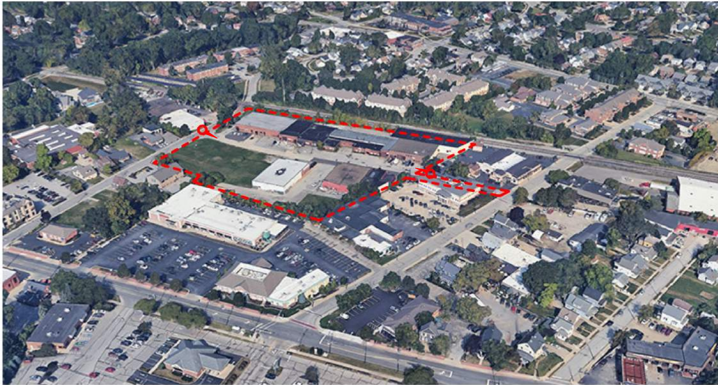
Aerial View of Site from the Southeast
