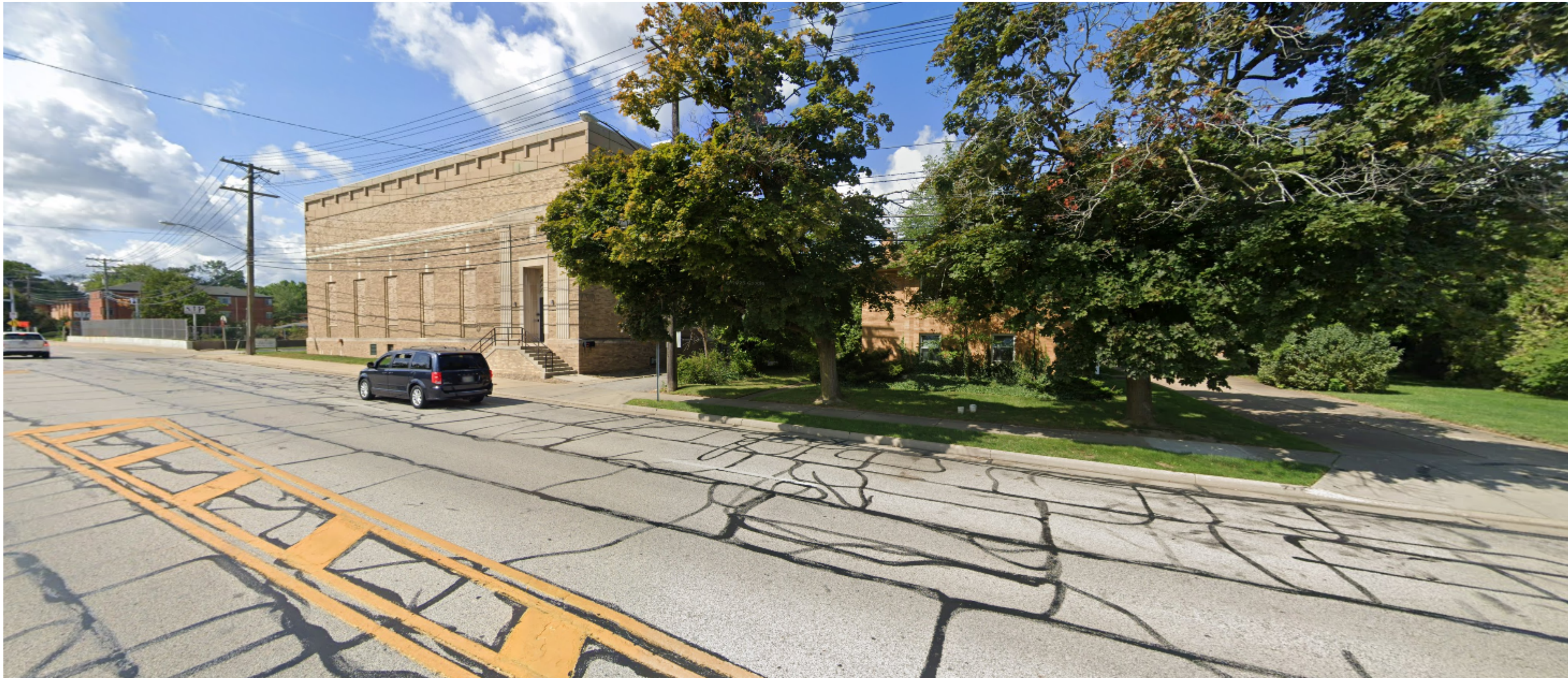
South - 1588 Wagar - Ohio Bell Telephone Bldg
